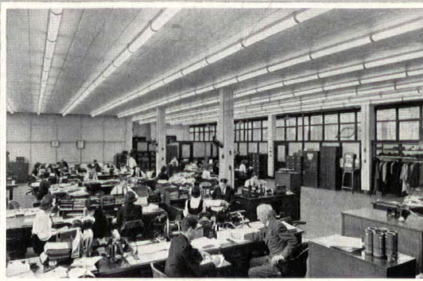
CL-40 fluorescent luminaires, ceiling-mounted in continuous runs, provide 40 to 45 footcandles of cool, shadowless illumination in this large industrial office.
