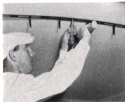
Strong, rigid prongs on ceiling runner are long enough to take care of variations in ceiling height.
