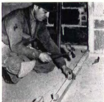
Metal Base Clip being applied to wood "sleeper," providing nailing base for wood trim. Or, clip can be nailed directly to concrete.
