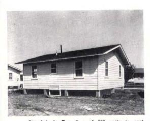
San Antonio, Tex. One of 300 units to cost \$814,000 plus a \$38,000 fee for local Contractor McKensie Construction Co. Unit cost: about \$2,800. Wire mesh is stretched between the concrete piers.
