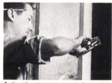
4. For side-wall insulation, staple flange of Masonite Cell-U-Blanket to face of studs, using ¼inch-long staples spaced not more than 6 inches o.c.
