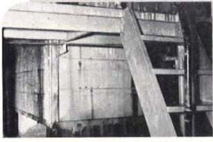
Wolmanized Douglas fir stock head-box, platform, stairs and rails in a paper mill.
