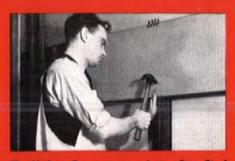
The Nailing Groove—an exclusive Stran-Steel feature—is one of the secrets of the fast erection of buildings framed with Stran-Steel. In the photo above, wallboard is nailed to the Stran-Steel studs. In the lower photo, corrugated sheet for a subfloor is being nailed to the Stran-Steel joists.
