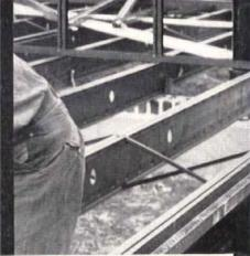
Assembling the Stran-Steel frame of an apartment building. Studs and floor joists are spaced 24 inches on center. Self-threading screws are used to hold the studs securely to the top and bottom plates. Note Stran-Steel method of lock-bridging between floor joists in background.
