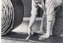
**2.** Cut Masonite Cell-U-Blanket 3¼ inches longer than the dimension between top and bottom plates, using sturdy scissors or spina.
