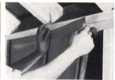
3. Then cut casing approximately 2 inches on both sides, fold back the Cellufoam core. Apply by stapling vapor barrier flange to face of plate.
