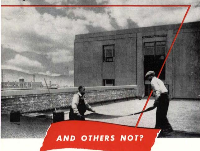
Why does one type of built-up roof last longer than practically all others? The reasons are pretty involved, but they all boil down to this simple fact: Coal tar pitch and tar-saturated felt are remarkably resistant to the disintegrating effects of sunlight and water.
