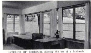
INTERIOR OF BEDROOM, showing the use of a fixed-sash "picture" window flanked on each side by Andersen Horizontal Gliding Window Units.
