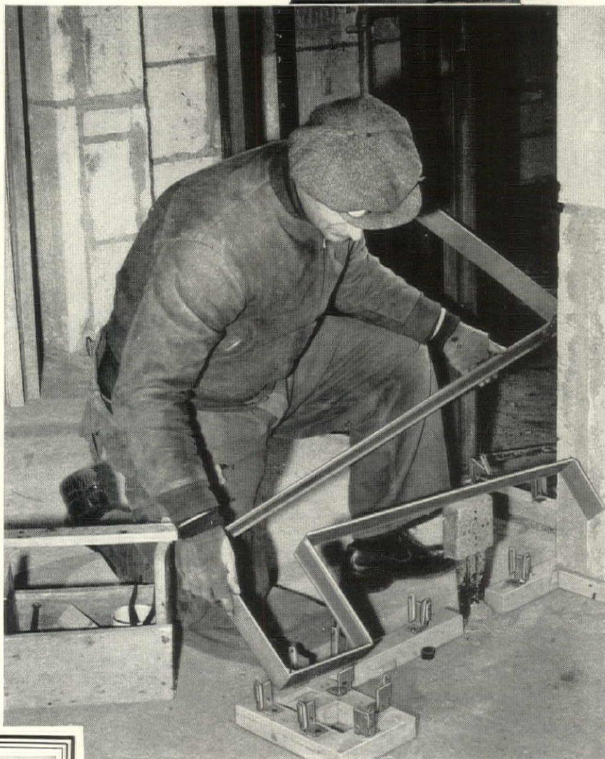
THE SECRET'S IN THE METAL BASE! The exclusive new metal base of the Gold Bond 2" Solid Partition System eliminates the need for prefabricated units. Base can be quickly cut and bent on the job to fit difficult angles and complicated conditions.
