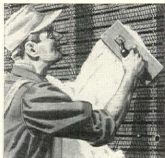
METAL LATH for elimination of plaster cracks, greater fire resistance. Partitions can be built of 2-inch thickness, saving space and considerable money on big jobs.
