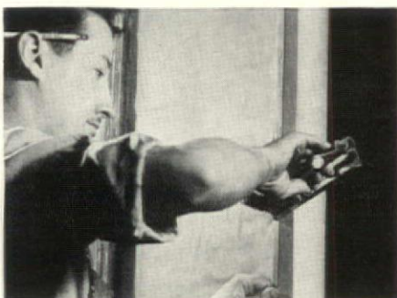
4. For side-wall insulation, staple flange of Masonite Cell-U-Blanket to face of studs, using \frac{1}{4} -inch-long staples spaced not more than 6 inches o.c.
