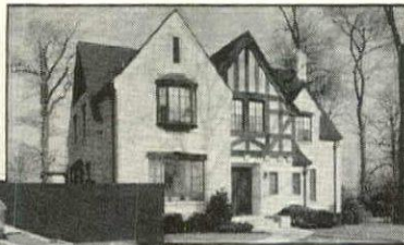
Dual-controlled, continuous circulation makes this system especially desirable in the multi-unit buildings.
