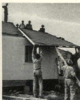
tion: 261 units. Subsequent Government contracts: 500 units. Photos show demounting, trucking and reerection of one-family
