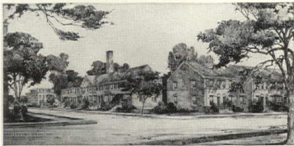
Carrollsbury Dwellings, the Alley Dwelling Authority, Washington, D. C. Francis P. Sullivan, Architect. 314 units in all. Each building has Bruce Streamline floors.
