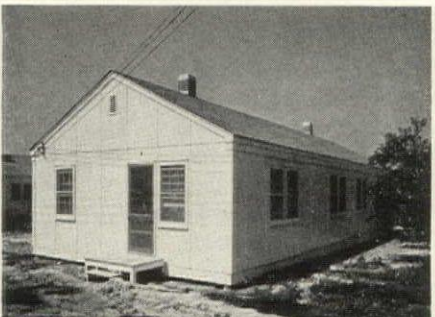
Plywood outside, plaster board inside steel frame at $2,295 for 16 singles, 54 doubles by Harnischfeger Corp., Milwaukee, Wis. Prior production: 400 units.
