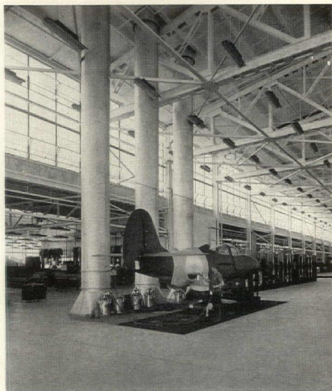
Open spray booth is ventilated with three fans which draw fumes from the paint guns down through a floor grille and exhaust them through the roof. Together, these fans move 45,000 cfm. Note that about half of the glass in the clerestory strip window is set in movable sash. Concrete floor has metallic hardener on surface.
