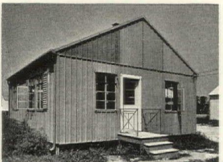
Steel outside, plaster board inside of steel frame at $2,770 for 10 singles, $2,796 for 48 doubles by Tennessee Coal, Iron & Railroad Co., Birmingham, Ala. Prior production: 1,460 dwelling units, 643 other buildings.
