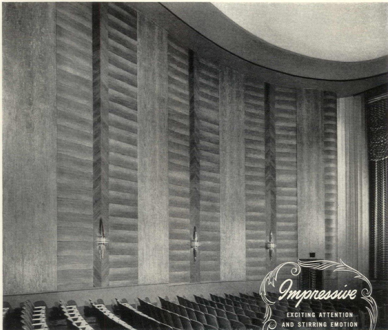
Honduras Mahogany and Ribbon Mahogany Flexwood treatment, Auditorium, Gladmer Theatre, Lansing, Mich., C. Howard Crane and Associates, Architects. Flexwood was used in several other theatres in the Butterfield chain.
