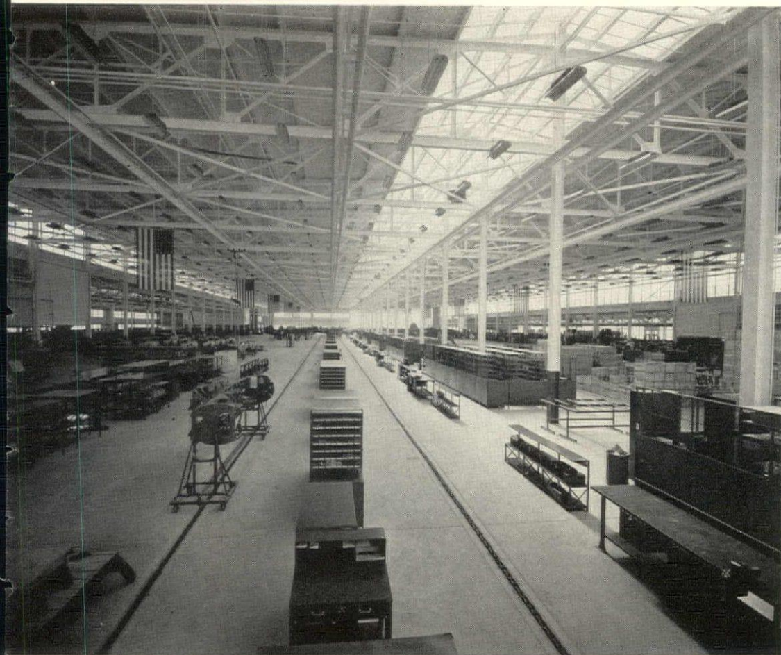
Final assembly area is divided down the center by a row of supporting columns. Each half is equipped with three conveyor lines, two of which are apparent in the view above. Parts bins separate the lines, permit mechanics to remain at their stations, concentrate on their repetitive operations while the planes are dragged slowly by. Note skylight running down center of entire plant and silhouetting one of the sixteen rows of fluorescent fixtures in the final assembly area.
