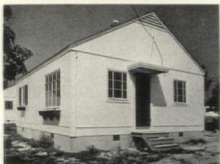
Plywood on wood frame at $2,976 for 39 singles, $2,981 for 24 doubles by National Homes Corp., Lafayette, Ind. Prior produc-
