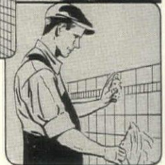
3. Joints are waterproofed and painted in matching or contrasting colored grout to make a beautifully finished job.
