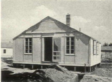
Plywood on wood frame at $2,988 for 23 singles, 43 doubles by Sears, Roebuck & Co. and General Houses, Inc., Chicago, Ill. Prior production: "thousands" by former; "several hundred" precut by latter.
