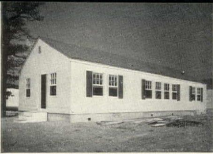
Plywood on wood frame $2,531 per unit for 10 singles, 40 doubles by Home Building Corp., Kansas City, Mo. Prior production: just a "few."
