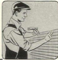
1. Foundation sheet applied over present walls—insulates and deadens sound.
