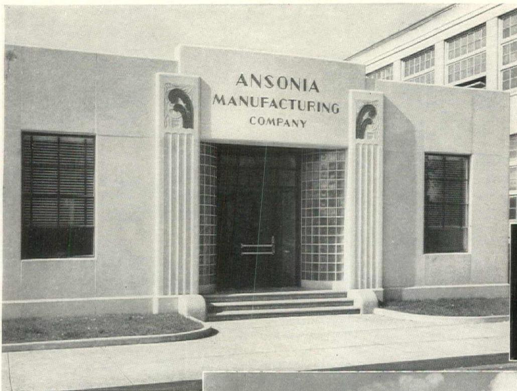
**OFFICE BUILDING**—Ansonia Manufacturing Co., Ansonia, Conn., faced with thin, precast Architectural Concrete Slabs. Use of slab as the exterior and bottom form for the structural lintel is shown in the detail. Note the size of this slab, 14'6" long by 6'1½" high. The company name and the design at top of each fluted column are of black aggregate and were cast into the slabs during fabrication. Architect, Brown and Von Beren; Slabs by the Dextone Co.—both of New Haven.
