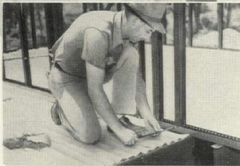
Studs are secured to bottom plate with self-threading screws. Notice that studs (and floor joists) are placed 24 inches o.c. This wide spacing is possible due to the great strength of Stran-Steel—results in savings of material.
