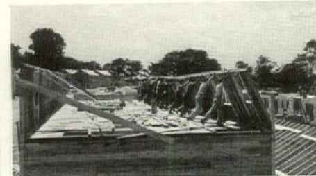
An entire wall for the second story of a four-family building goes up with a push by a score of workmen.
