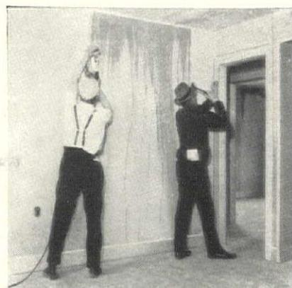
Sanding off glue at joints of Mengel Bord, and applying trim before papering and painting.
