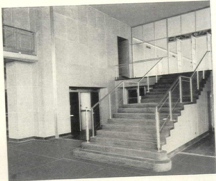
**SLABS FOR INTERIORS**—Washington National Airport. Attractive texture of exposed aggregates in an almost infinite variety of colors and patterns is a feature of thin, precast slabs. Texture may be pre-inspected. This interior is of buff quartz aggregate embedded in a matrix of Atlas White cement. Architect, H. L. Cheney, Washington; Contractor, John McShain, Inc., Philadelphia; Slabs by Dextone Co., New Haven, Conn.
