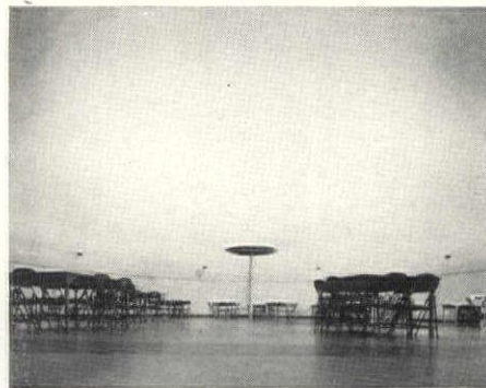
Lighting for the main dining room is provided by a single, centrally-located fixture 8 ft. in diameter and 12 in. deep.
