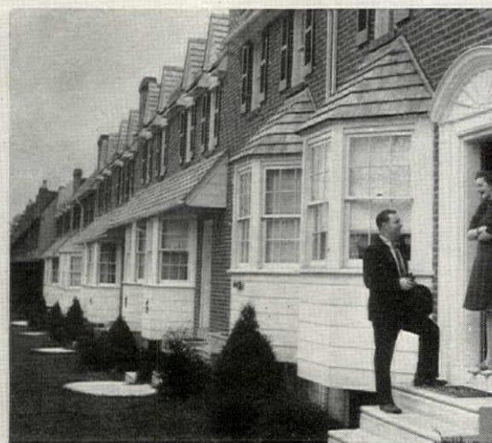
Norge Model OB-60T was the standard heating plant in 196 row houses in the McClatchy Subdivision, Upper Darby, Pennsylvania.
