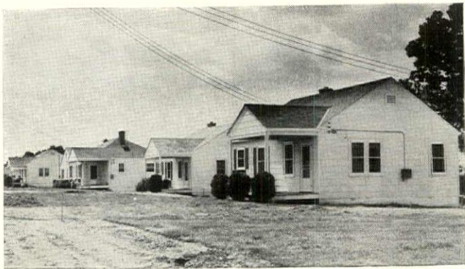
Section of Tremont Gardens Development at Falls Church, Va., which is now using "Pyrofax" Gas.
