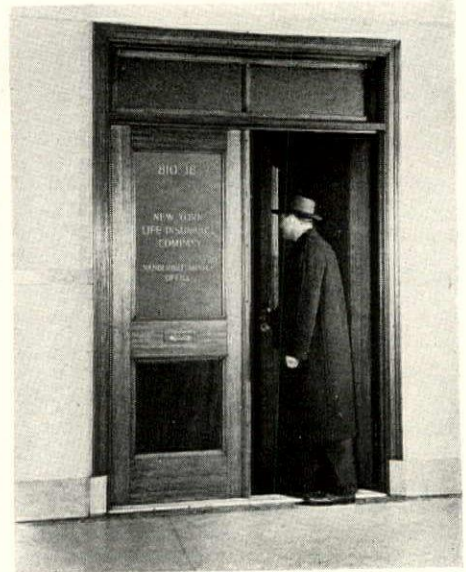
Glass was removed from corridor doors within safe areas, replaced with non-shattering fibre board panels with duplicate of tenant's sign in gold leaf.
