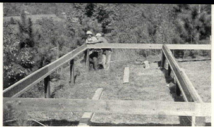
Foundation posts for the minimum defense house are wood posts, designed to last 8 or 10 years in most soils.
