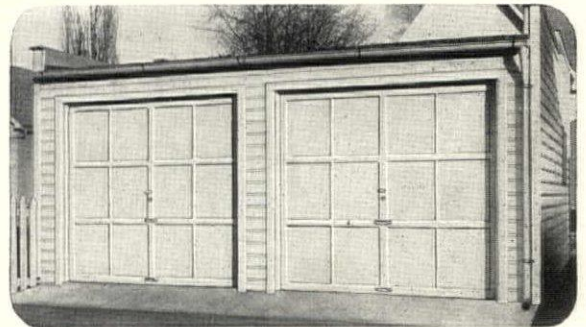
Installation of Ro-Way Model "R" Overhead Type Doors in 2-family residence garage.
