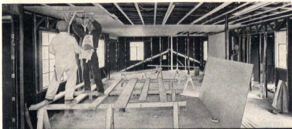
Immediate application of panels follows enclosure of building. Upson Floating Fasteners on either steel or wood framing, grip panels from the back, allowing normal structural movement.
