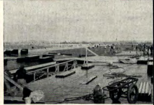
As soon as the first area of Q-Deck is laid, the application of insulation and waterproofing is carried on concurrently, thus making speed.
