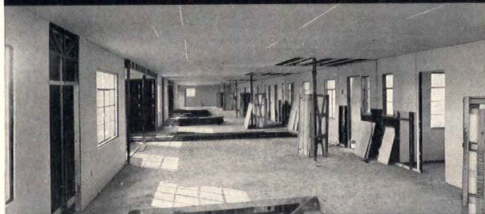
Walls and ceilings of a typical five-room house have been finished in as little as 40 man-hours. 100% salvage in demountable units is possible.
