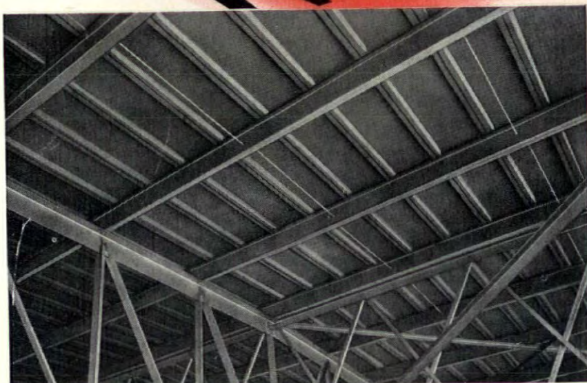
Showing the smooth, finished ceiling effect provided by the underside of the roof slabs.
