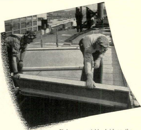
Slabs are quickly laid on the roof purlins in any weather. Occupant can get under cover and into production, fast.
