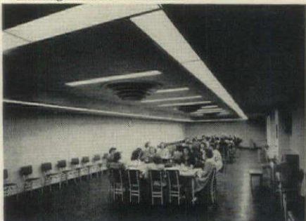
★ The Basement Lunch Room and Recreation Area gets 50 footcandles from its 56 Troffers arranged in a rectangle.
