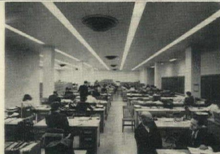
★ In the General Office, continuous Troffers, covered at the bottom by Satinol Flurex glass (as are all the Troffers throughout the installation) provide 50 footcandles in service.
