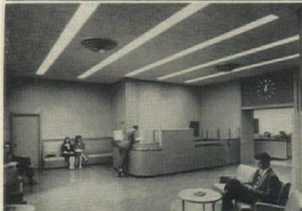
★ The Foyer is lighted by 5 rows of Troffers, on 50-foot centers. Fifty to 55 footcandles is maintained to create a cheerful, comfortable atmosphere for those awaiting business conferences.
