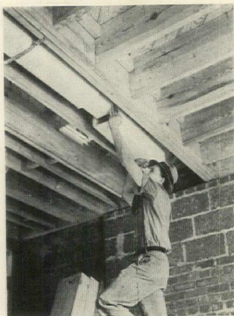
2, All-Asbestos Duct Saves Steel for War
