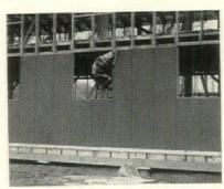
For Outside Walls—Gold Bond Exterior Board which comes with tough asphalt roofing on the weather side. Takes care of sheathing and siding in one operation, building sturdy permanent walls with saving in time and money.
