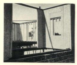
Above, Armostone system, a single-wall, precast system employing channel-shape units to form concrete studs. Below, the Simpson Craft system, which used flanges of precast wall panels as a form for cast-in-place studs.
