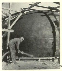
Final stages in the construction of the Neft "bubble" house (see also pictures on preceding page). 4. shows workman applying first "Gunite" coating, which was followed by insulation and a layer of waterproofing, shown being applied in picture 5. Views 6. and 7. show almost-completed and completed houses, which consisted of two such dome-like units separated by a connecting link of conventional block construction.
