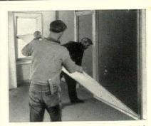
For Inside Walls and Partitions — Gold Bond Solid Partition Panels are fastened between the study by mouldings. Their large size means speed on the job. Their strength insures solid, rigid walls. Permanent or demountable and completely salvageable.
