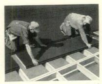
For New Roofs or Roof Repairs—Gold Bond Roof Plank is a heavy, durable gypsum board, which nails directly to wood joists and is quickly applied by any carpenter. Perfect base for built-up roofing. 1½" and 2" thick, 24" wide and 8', 9' and 10' long.
