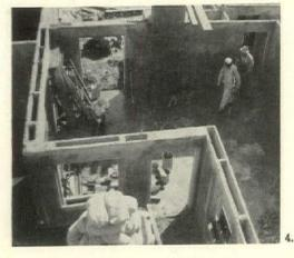
Hayes "Econocrete" system of cast-in-place construction. 1. shows sectional exterior form, 2. room-sized interior form. 3. is a "cut-away" set-up of the typical wall, showing hollow core and method of reenforcing and installing pipes and wires. 4. shows section of completed walls.
