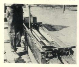
Below are two views of the process of construction developed by John J. Earley, Washington, D. C., "craftsman in concrete" in 1935. Earley's precast panels were faced with decorative, crushed-stone aggregates, attached to a wood frame to which conventional interior finishes were applied.
