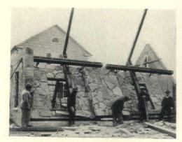
Above, Carroll "Tri-Ply" method of monolithic wall construction. Rock faced panels were cast on the floor, raised into position with a special hoist. Picture below shows apparatus for casting double monolithic walls according to the Van Guilder system, using a collapsible metal form.
