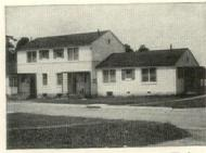
One of 300 houses for war workers at Hatboro. Pa., finished with white-cement paint made with Atlas White cement. Maintenance cost for these homes will be low because the white-cement paint provides a protective covering. Good-Looking Finish Ideal for Housing and Other War Structures Easy to Mix and Apply . . . Uses No Critical Materials
