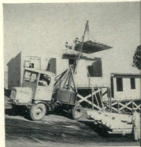
Application of Homasote "Precision Built" system of prefabrication (Barrett & Hilp, Builders) in war housing. Pictures at top of page show shop assembly, on jig tables, of wall and roof panels, middle picture job assembly of floor panels, bottom picture truck-crane lifting roof panels in place.
