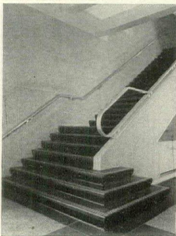
Fine Terrazzo is used in this hospital for floors, walls and stairway. Stair treads and risers are of precast terrazzo. V. Foscatto Inc., Long Island City, N. Y., Terrazzo Contractor.
