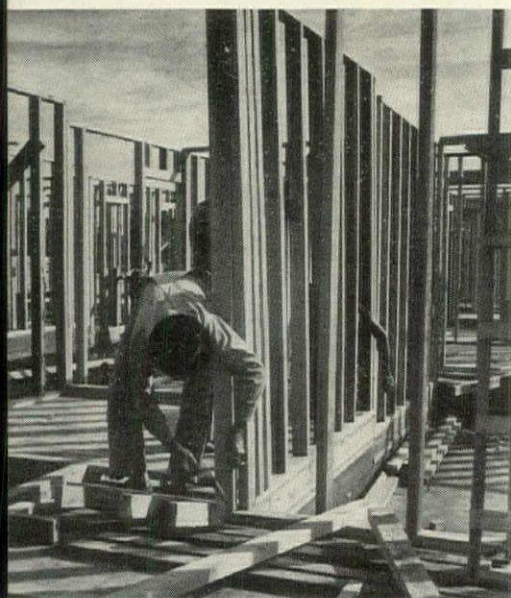
Various stages in a system of precutting framing lumber to individual house plans, worked out by Builder Paul de Huff in 1938. Top picture shows special saw table with spacer tabs which permitted simultaneous cutting in various lengths, middle picture packaged members ready for trucking to the job, lower picture assembly of frame.
