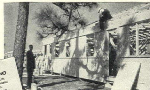
Cemesto construction is sturdy and economical. Houses are finished at the rate of 20 a day.
