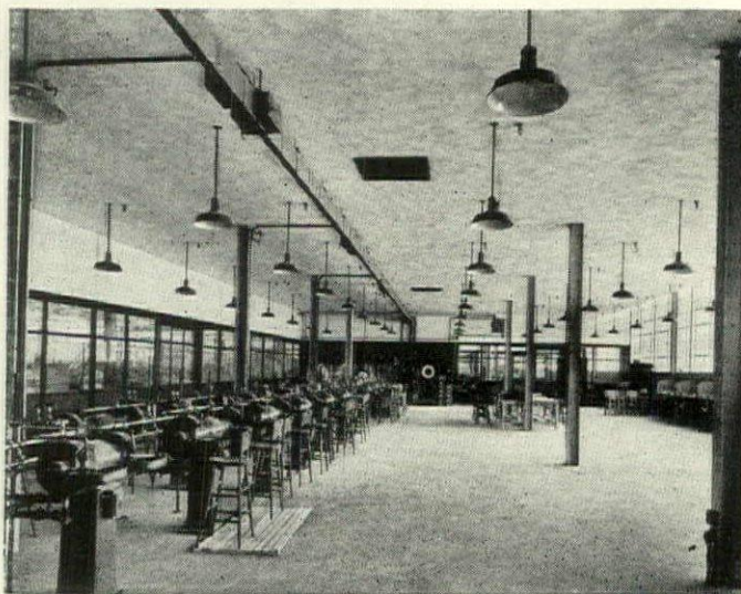
ONE OF THE GRINDING ROOMS. Because of the specialized nature of this operation, the department is partitioned off from the remainder of the plant. The ceiling is plastered over, rather than left open with exposed trusses, to prevent the collection of dust.
