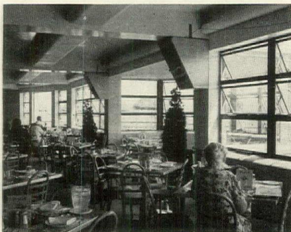
MUSIC FOR A RESTAURANT is projected through wide-range loud speakers on columns. These Western Electric speakers are actually two units—one transmitting high frequencies and the other low frequencies. This installation was planned by the Langevin Co.
