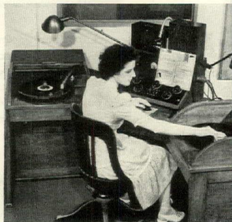
CENTRAL STUDIO of the Muzak Corp. in New York City. Dual turntable permits continuity of music programs. Operator follows program sheet on control panel and monitors with volume control indicators.
