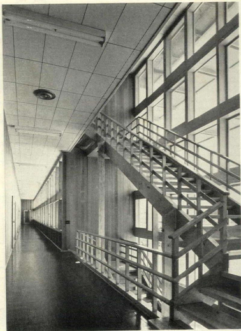
THE MAIN STAIR: A FINE DETAILING JOB USING STOCK MATERIALS
