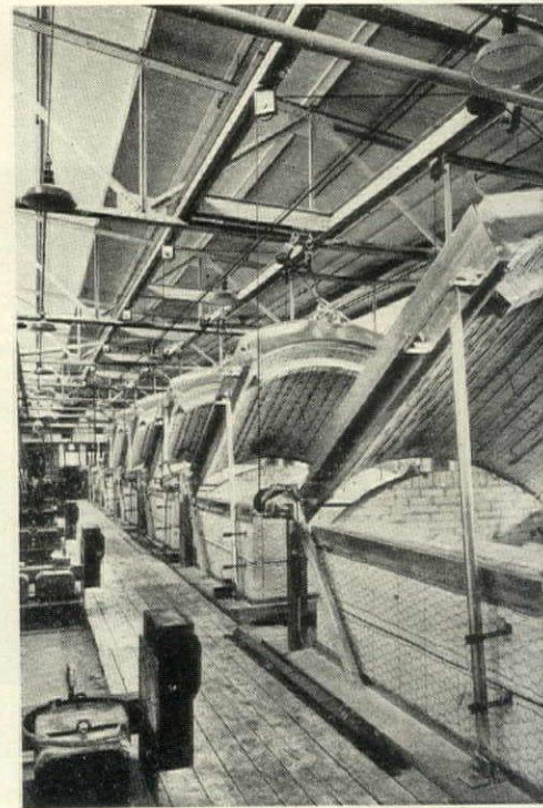
FINAL ANNEALING KILNS , used for cooling after the second melting. Tops of kilns are raised and lowered from supports on the structural steel trusses above.
