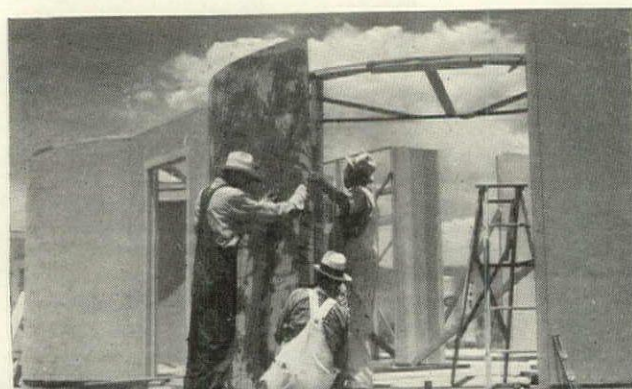
IN SECOND HOUSE, THE SHEETS WERE BENT IN PLACE
