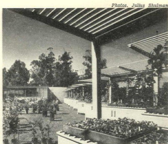
PLANT BARS ARE STAGGERED, BUILT OF WOOD
