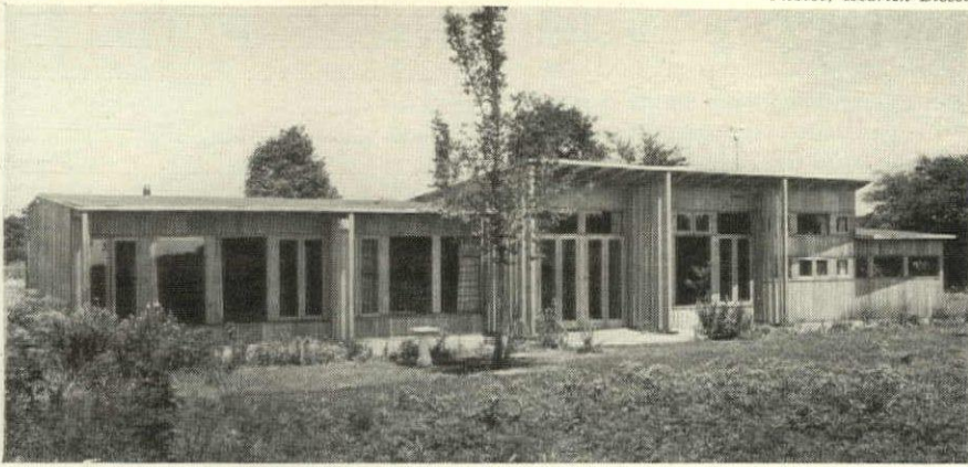
TEST HOUSE is oriented with large windows along the entire south side. In summer, wide projecting eaves prevent the sun from entering the building.
