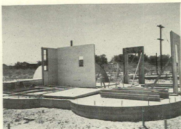
PANELS PARTLY UP. ERECTION TOOK THIRTY HOURS
