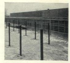
Monarch Machine Tool Company, Sydney, Ohio, needed a sizable addition to their plant by April 1. Work started January 17. The contractor chose Atlas High-Early cement. Mean temperature during concrete placement stayed below freezing—fell as low as 10°F. Concreting was completed thirteen days ahead of original schedule date.
