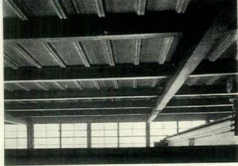
ROOF STRUCTURE IS COMBINATION STEEL AND CONCRETE
