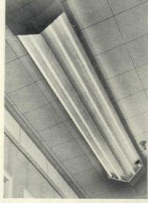
FIXTURE contains four 8 ft. lamps for high-level illumination in an office of the Higgins Shipyards in New Orleans.
