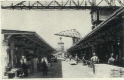
2 MACHINE PRODUCTION—"Assembly line" production methods with specialized equipment enables the Henry Mill to fabricate heavy timber structures faster, cheaper, and with greater precision than is possible with hand-framing methods.
