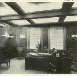
RECESSED TROFFERS in ceiling form attractive pattern, provide efficient light without glare. Glass panels diffuse the light and improve its distribution.
