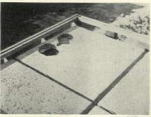
KNOCKOUT holes for plumbing connections are provided in duplicate for use in left-hand and right-hand plans. Unused hole is filled with cement.
