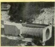
II ft. diameter axial-flow fan with exbaust stack and air shaft bood delivering 500,000 CFM at 6½" static pressure.
