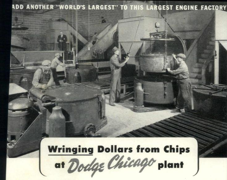
FROM THE WORLD'S LARGEST line of machine tools, in the world's largest aircraft engine plant, come thousands of tons of chips and turnings. Dripping with machine cutting fluids, they are literally worth their weight in gold—in reclaimable oils and metals.
