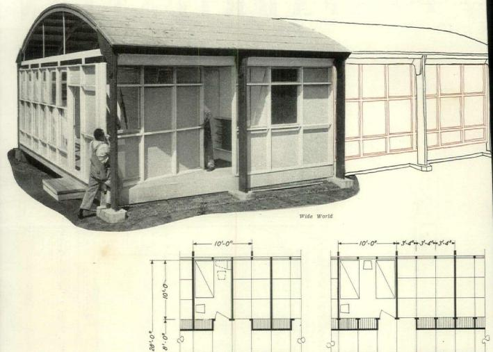
can be inter-changed and moved about even after the building is complete, and puts the structural frame-a series of free standing posts-on the outside of the building. To replace the conventional gable roof, supported by triangular trusses or rafters, it employs a remarkable arch roof in which curved, standardized panels are put together like bricks to form barrel vaults spanning the entire width of the building.
