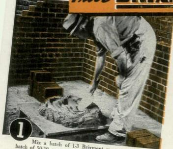
Mix a batch of 1-3 Brixment mortar (above) and a batch of 50-50 cement-lime mortar made with the same proportion of sand (right). Get any competent bricklayer to test
