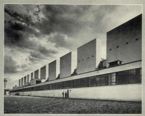
Characteristic structural unit for virtually the entire plant is the reinforced concrete arch roof.
