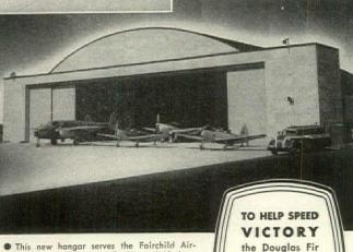
● This new hangar serves the Fairchild Aircraft Division of Fairchild Engine and Airplane Corporation. Eight 17' x 27' Exterior-type Douglas Fir Plywood doors designed by Fairchild engineers cover the 136' x 27' portal.
