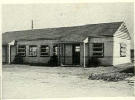
THIN CONCRETE slabs form walls of these small houses. New method of electrical prestressing is quick and accurate. Thermoplastic-coated bars are heated, nuts on threaded ends are taken up; when bars cool, coating restores bond. After three or four days, 21/2-in.-thick walls are lifted into place.
