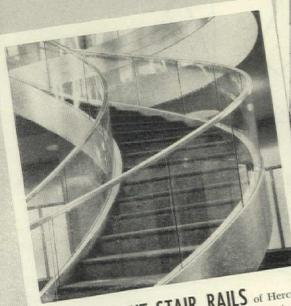
TRANSPARENT STAIR RAILS of Herculite Plate Glass offer new design possibilities both in public building and residential interiors. Herculite Glass is tempered to give it approximately 4 times the strength and 6 times the impact resistance of normal plate glass. Architects: Reinhard & Hofmeister and Harrison & Fouilhoux.
