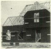
frame building... with Gold Bond Gypsum Sheathing. Lightweight panels of processed gypsum rock fit standard stud spacing. Can be sawed like lumber for the little trimming needed. Rock-like construction adds greater strength to the building.
