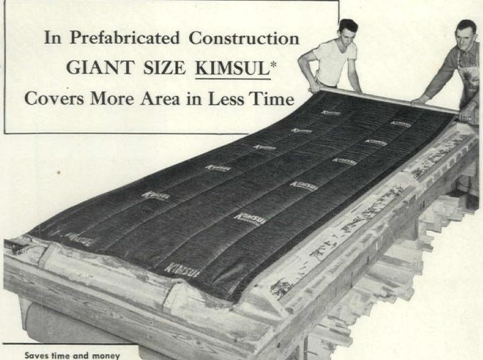
Picture above shows how KIMSUL blanket covers prefabricated ceiling panel in one operation. Floor panels are insulated similarly; flooring is nailed right over the insulation.
