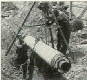
Section of Ric-wil prefabricated insulated steam conduit being lowered into shallow trench for steam connection to a new apartment at Shaker Square.
