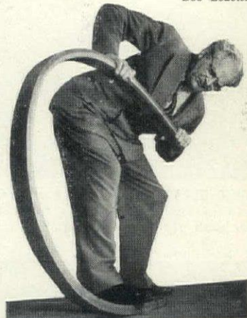
"COMPREG" may also be bent by hand. Impregnated and compressed, this product has strength as yet unknown in wood.
