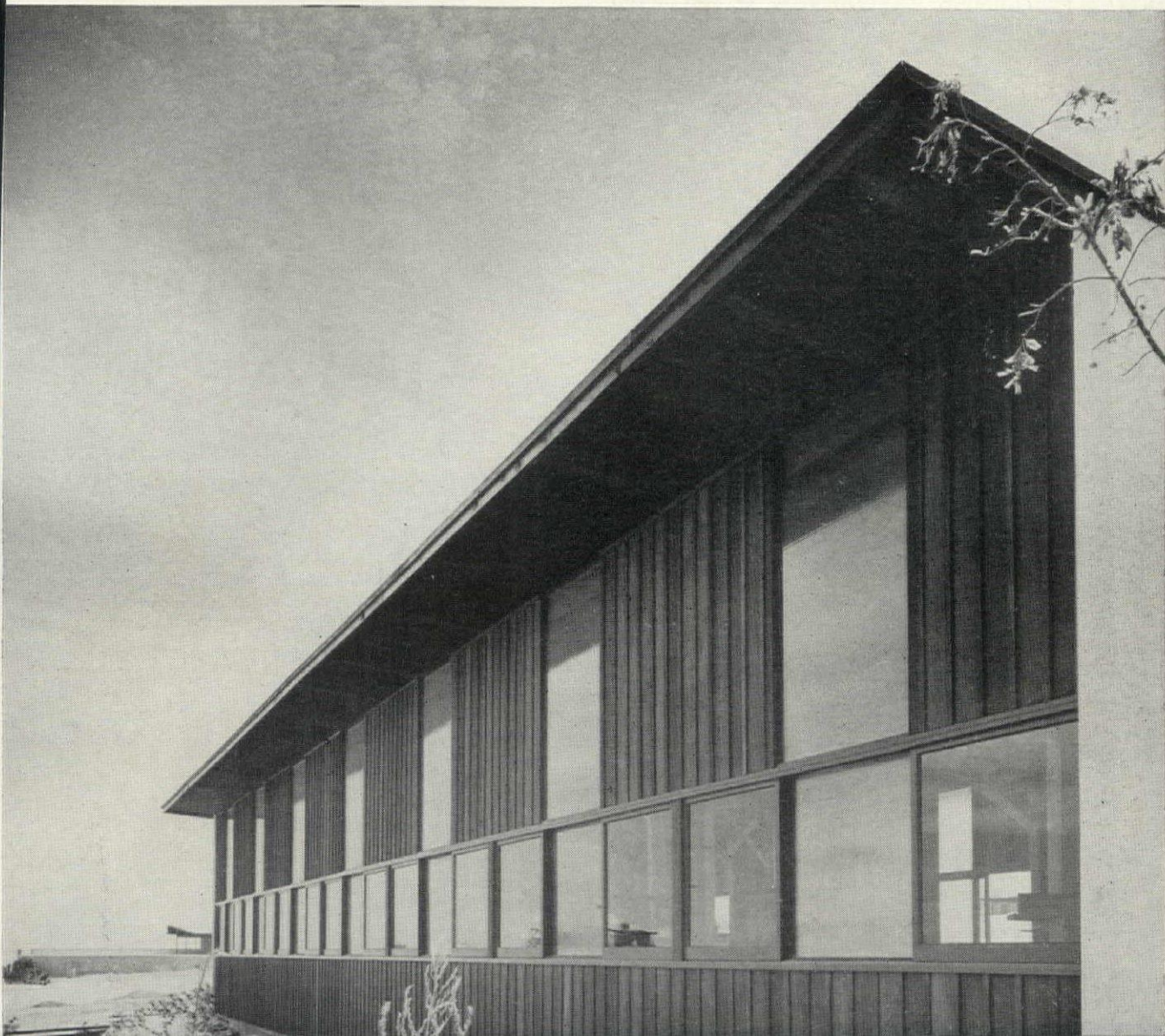
SERVICE BUILDING SHOWS FREEDOM POSSIBLE WHEN EXTERIOR WALL DOES NOT SUPPORT THE ROOF
