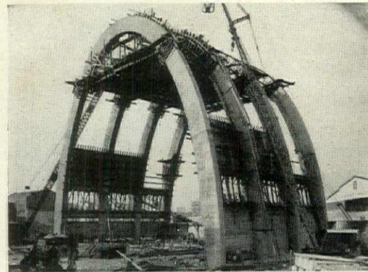
LIGHT STRUCTURAL STEEL members were used for reinforcing and as support for the forms. Sides of ribs were grooved for installation of barrel walls, which were formed with wood for interior face and long pine planks for exposed surface.
