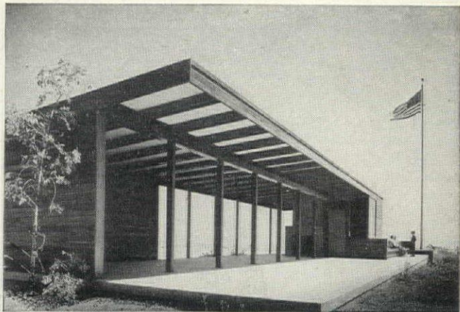
GARDEN CRAFT BUILDING: EXPOSED ROOF STRUCTURE IS USED AS A MAJOR DECORATIVE ELEMENT
