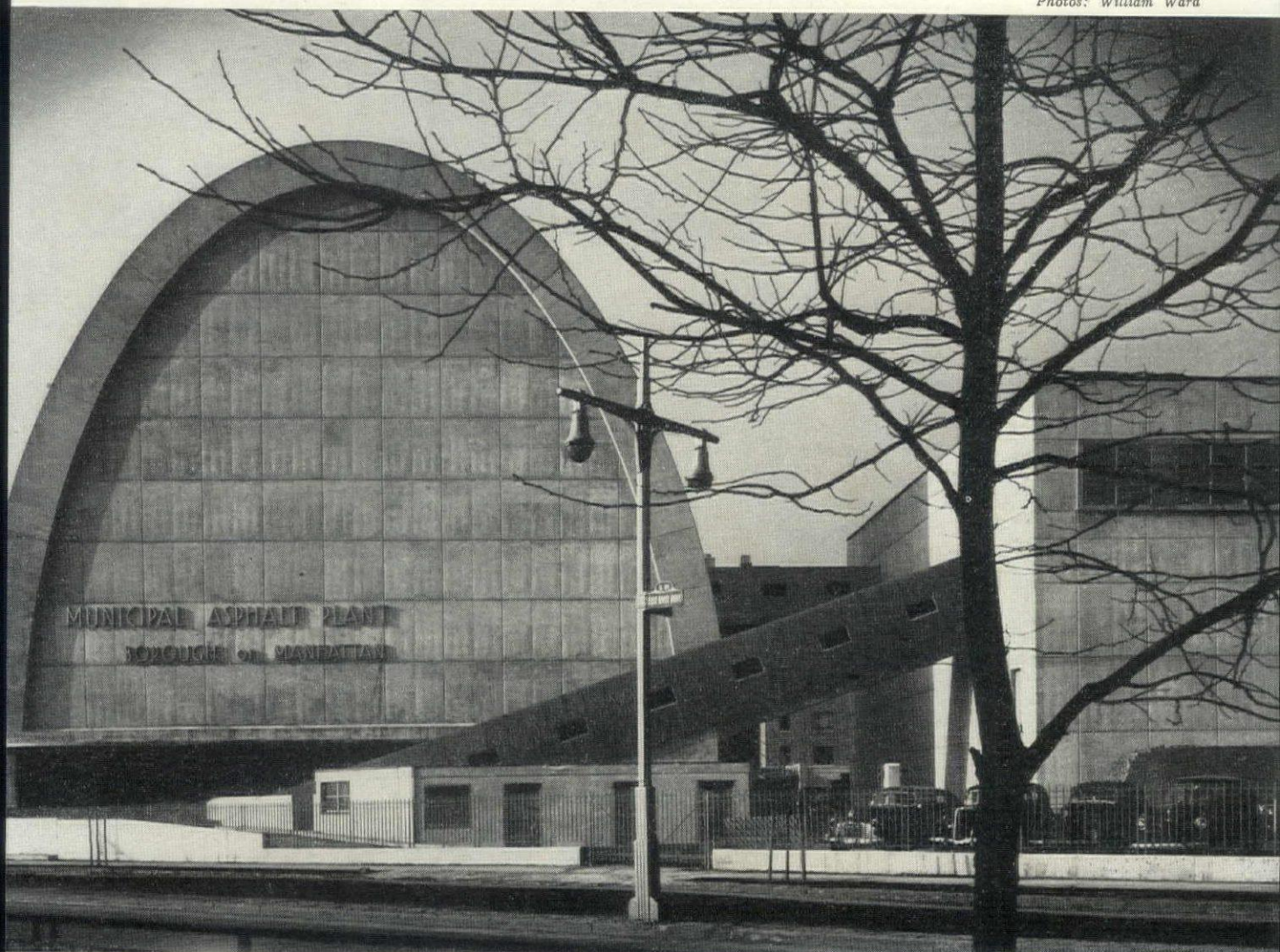
AL ARCH CONSTRUCTION ELIMINATES NEED FOR HORIZONTAL BRACING REQUIRED BY RECTANGULAR SHAPE
