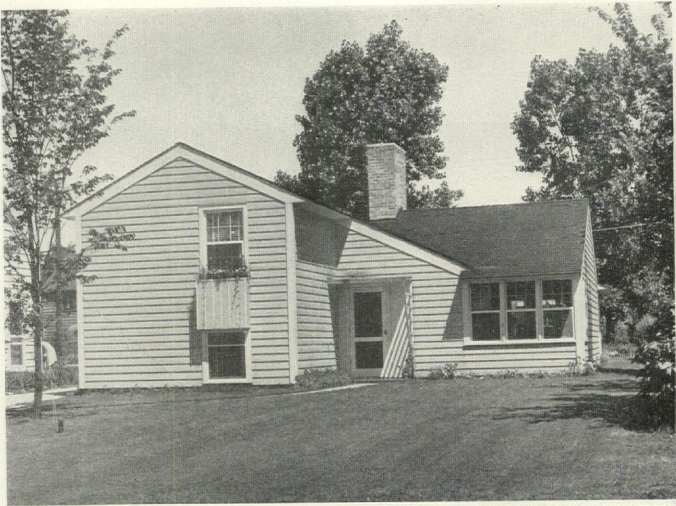
FRESH HANDLING OF TRADITIONAL DESIGN ELEMENTS. WINDOW GROUPING ELIMINATES THE NEED FOR SHUTTERS
