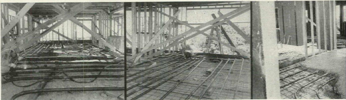
THREE PROGRESS PHOTOGRAPHS SHOWING SUCCESSIVE STAGES IN THE INSTALLATION OF THE HEATING COILS
