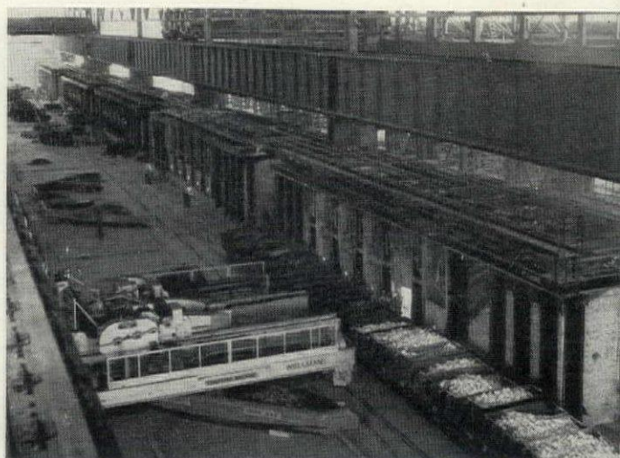
CHARGING MACHINE PUSHES MIXTURE INTO FURNACES
