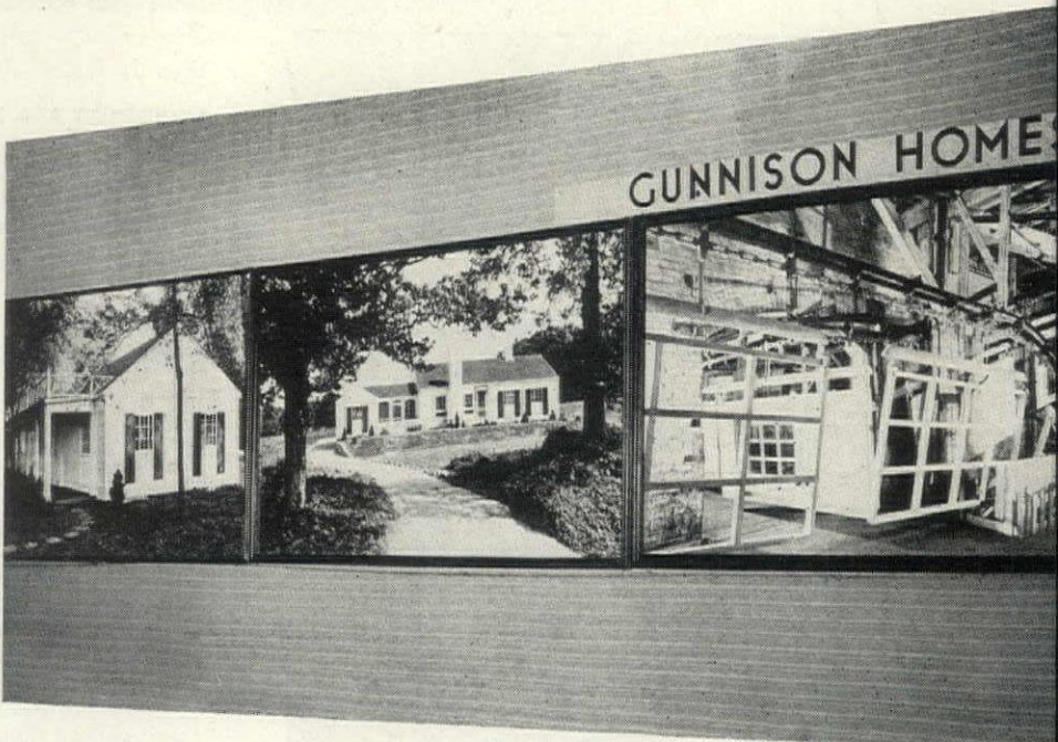
TYPICAL PREFABRICATED HOUSES and one interior view of the factory which is equipped to turn out a finished house every 25 minutes comprised the Gunnison Company's simple exhibit.
