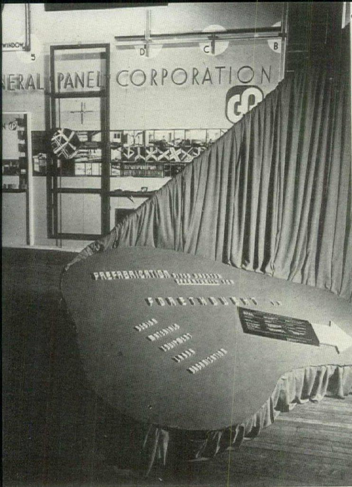
AMONG the exhibits was General Panel's graphic presentation of their prefabricated Packaged House, developed for them by Konrad Wachsmann and Walter Gropius. It consists of standard panels, completely equipped and finished, which act as both material and supporting elements for the building.
