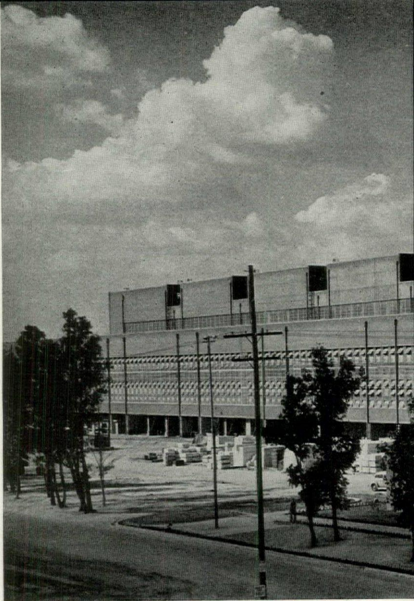
OPEN HEARTH BUILDING WHOSE FURNACES CONVERT PIG IRON INTO
