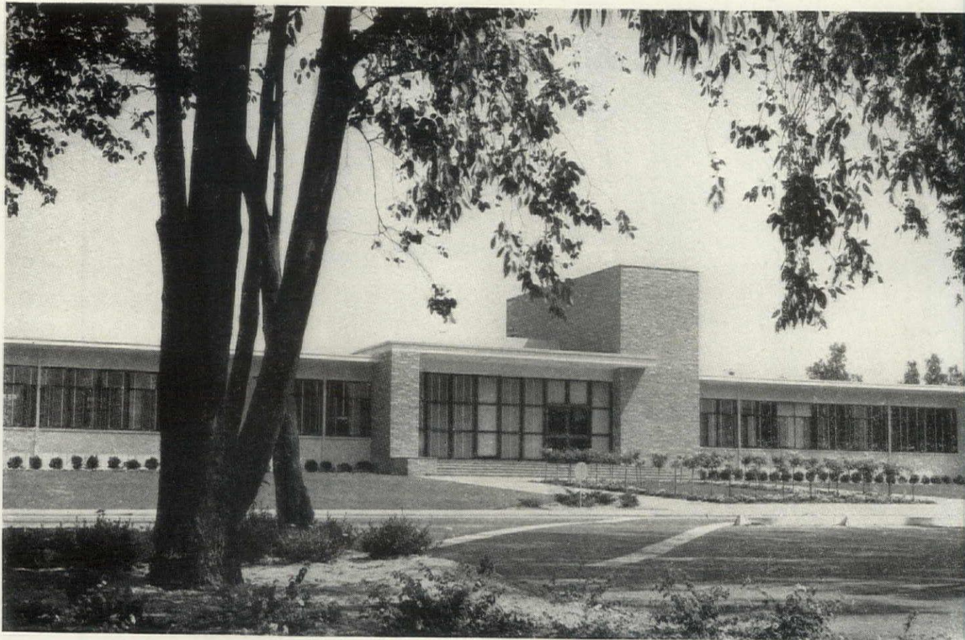
WINDOWS ARE UNINTERRUPTED BY STRUCTURAL COLUMNS, ROOF IS CANTILEVERED FROM CENTRAL CORRIDORS
