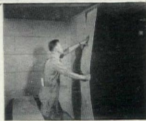
Next, spring Rocklath plaster base into ceiling runner groove.
