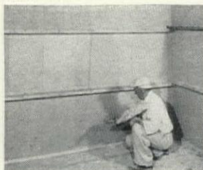
Both sides are plastered with scratch coat and allowed to set.
