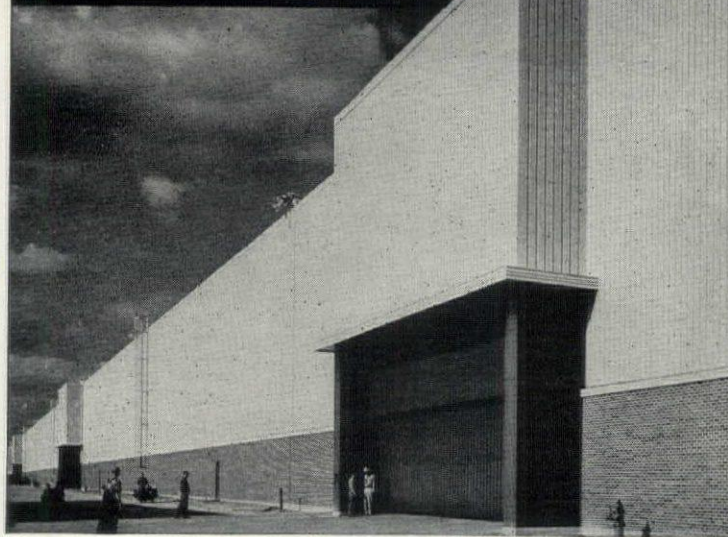
Windowless, completely air conditioned plant of Consolidated Vultee Aircraft Corp. at Ft. Worth, Texas, designed and built by The Austin Company. At right are some of the refrigerating compressors. Condensers are on level below.
