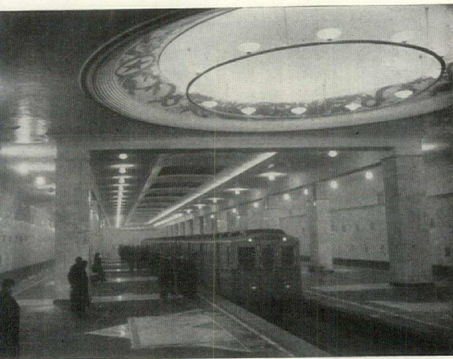
VENTILATORS LOCATED ABOVE TRACK MINIMIZE PLATFORM DRAFTS
