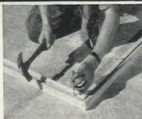
First, floor and ceiling runners are nailed securely in place.
