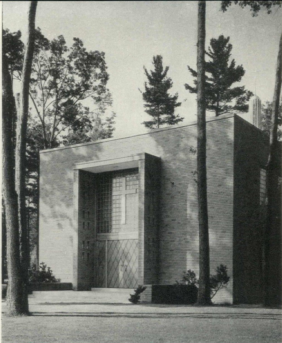
Photos: Ezra Stoller
