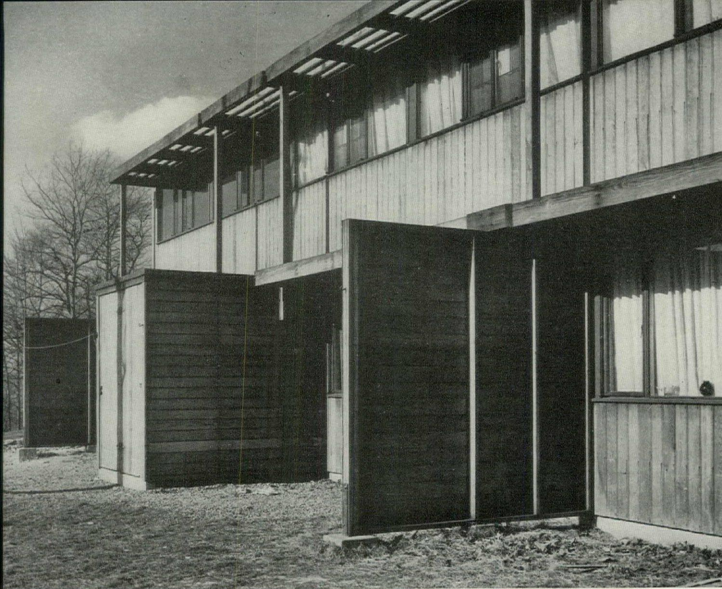
REAR OR "WORKING" SIDE OF 2-STORY, 8-UNIT ROWS IS BROKEN BY PROJECTING WALL PARTITIONS AND UTILITY S
