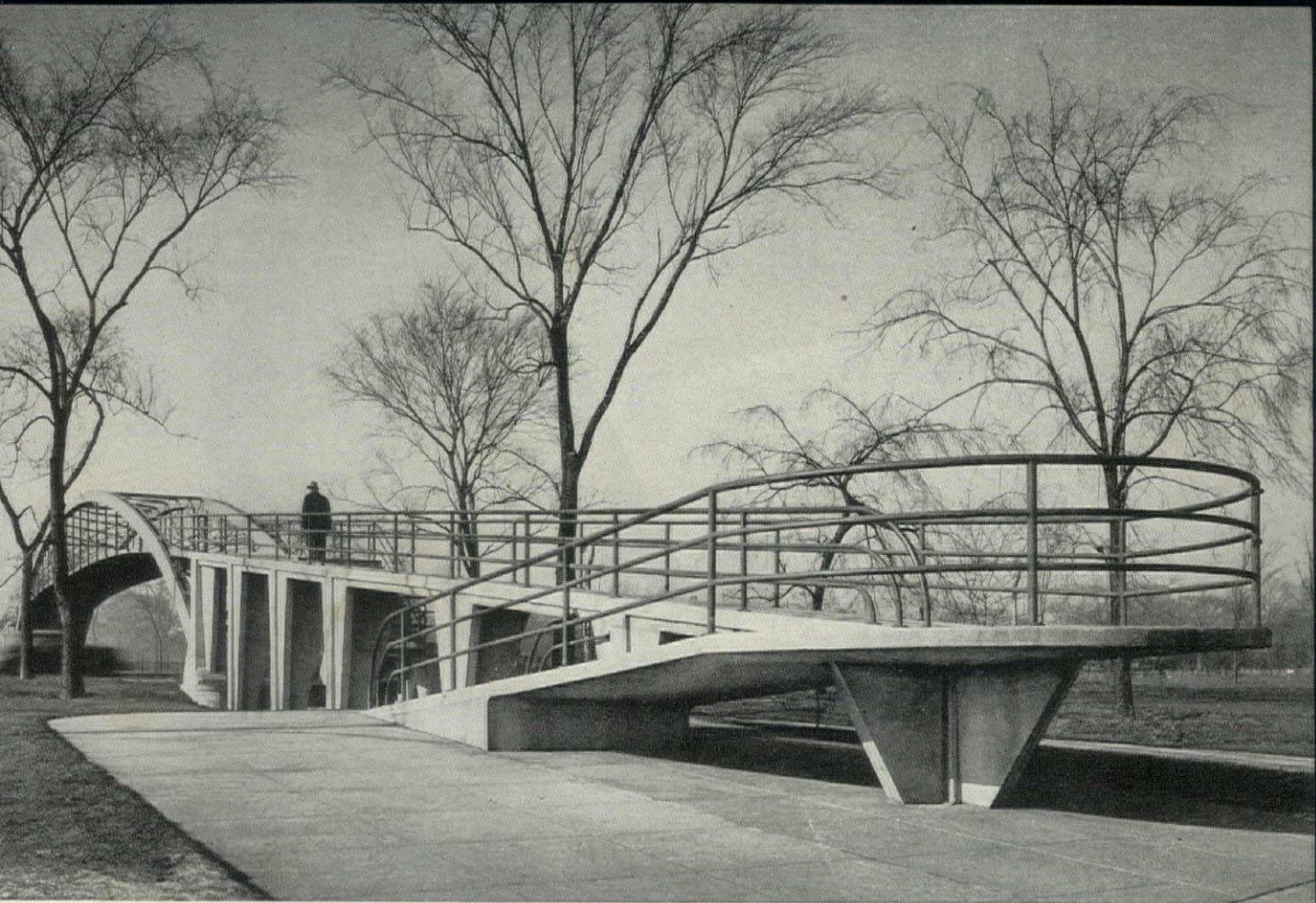
BRIDGE IS APPROACHED FROM BOTH ENDS BY LONG, CURVING RAMPS WHICH ACCOMMODATE BABY CARRIAGES AND BICYCLES
