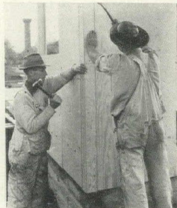
INSTALLING CORNER CASING
