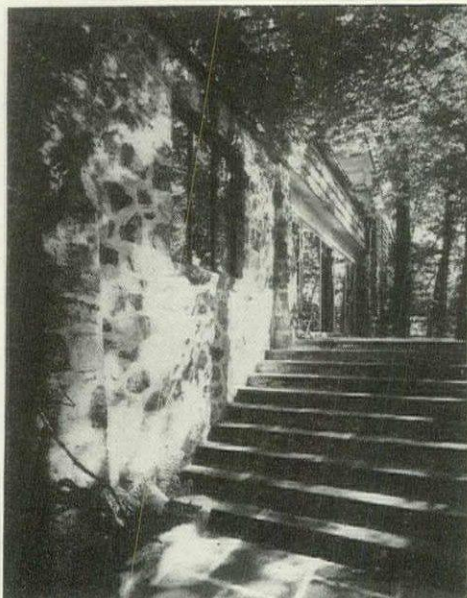
2. STAIR TO TERRACE AND ENTRANCE
