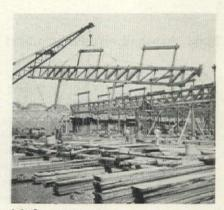
July 2 prefabricated truss sections including framing for monitors were erected.
