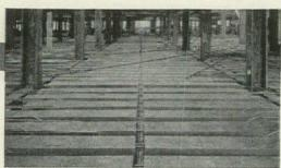
Eliminates extra framework . . With the Meyer Steelform you use a simple open wood centering, that can be removed and re-used with the Meyer Steelforms from one floor to the next.
