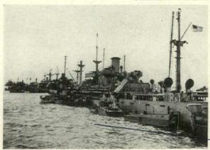
Sunken Liberty ships and other merchant vessels are used in combination with caissons to create a stout seawall. They are in turn protected by floating steel breakwaters anchored further seaward.
