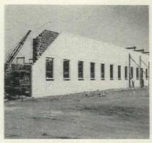
June 12 superstructure started. Photo shows the cavity type exterior block wall.
