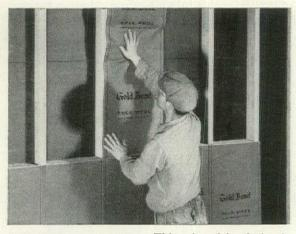
GOLD BOND ROCK WOOL. This mineral insulation is fireproof—not merely fire-retarding. Provides the maximum in insulating efficiency. New semi-rigid batts have more "body", are more easily applied.
