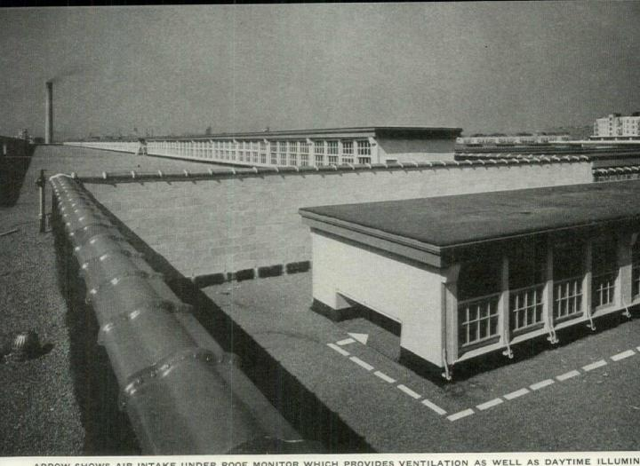
ARROW SHOWS AIR INTAKE UNDER ROOF MONITOR WHICH PROVIDES VENTILATION AS WELL AS DAYTIME ILLUMIN
