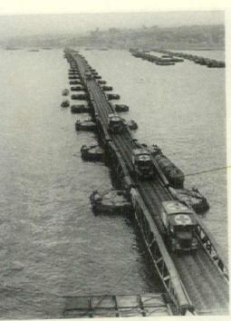
Prefabricated spans supported by pontoons create a floating causeway to reach off-shore piers in deep water.
