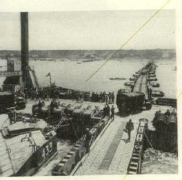
Ships are unloaded at concrete piers set parallel to shore line. These are linked together by short spans of roadway.
