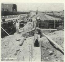
June 1 marked the beginning of reinforced concrete foundation wall construction.
