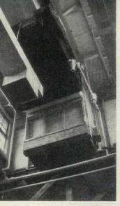
Wers in monitors draw 47,000 cu. r per hour into the structure in and circulate air heated by steam power plant in winter.
