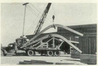
LAMINATED KNEE BEAMS, shaped to specifications for a chapel at Corvallis, Ore. were fabricated by Timber Structures Inc.
