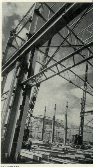
ALL-WELDED 65 ft. building columns for the Electro-Motive pi together with crane columns on either side, were fabricated in Austin shops as one piece. Each of the columns weighs about 8 ft.
