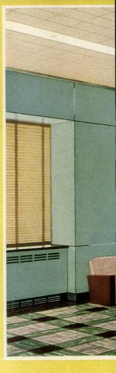
Movable Walls: J-M Transite Walls are strong, sturdy, durable. They provide a complete system of dry-wall construction, which can be taken down and relocated almost overnight with 100% salvage. Available for any heighteven for low railings and counters. Made of asbestos and cement, they have a smooth, hard surface. Fireproof. Last indefinitely. May be left in original gray finish, painted or decorated.
