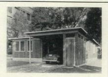
by registers cut into the floors. The 8 by 16 ft. prefab units are built from insulated panels framed by interlocking steel strips.
