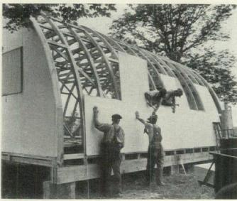
SMALL ARCHES in Purdue University research house are made of laminated wood, successfully reducing use of connectors.
