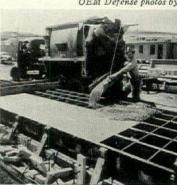
SIMPLE GRID FORM used for site p tion of poured concrete piers at \ Calif. turns out 84 in a single ope
