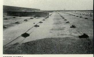
SPENT WATER from air-conditioning systems is sprayed on the of some controlled-conditions plants to help meet peak cooling to
