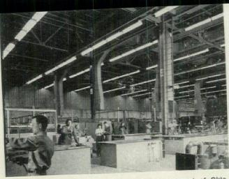
VENTILATING DUCTS in cadmium plating department of Oklahoma City plant eliminate the need for full-length partitions which would otherwise interfere with free-flowing production.
