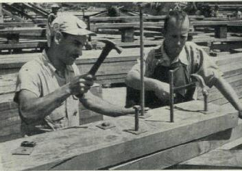
TIMBER TRUSSES for 246 ft. span Navy blimp hangar were fabricated by Timber Structures Inc. Connectors were made by Timber Engineering Co. Rings fit between members, are center bolted.
