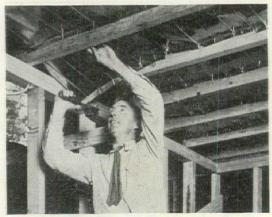
Ferro-Therm is stapled permanently in place; it cannot settle or pack down.
