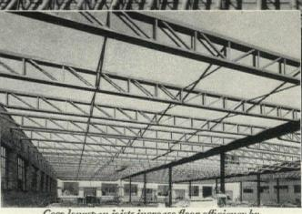
Ceco longspan joists increase floor efficiency by reducing number of columns.
