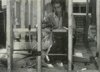
SARAN TUBING, an extruded plastic for hot and cold water plumbing, is extremely flexible, resists temperatures up to 170° F. and may be flared or bent. Top photograph illustrates tee, elbow and coupling connections, lower one shows installation. Fittings can be either plastic or metal.
