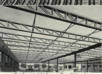
Ceco longspan joists increase floor efficiency by reducing number of columns.
