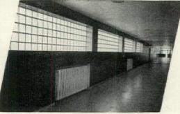
Panels of Insulux have been used to brighten the dark in corridors, stairwells and entry ways.
