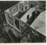
WALLS are placed in nine units. Picture at left shows living room wall 20 ft. long, 8 ft. high and  $2!_{2}$  in. thick hoisted into place in one piece. Material is resilient to allow handling of large units without cracking. In picture above sliding doors operate in a sheet metal channel.
