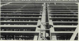
All Meyer Steelform construction requires is this simple open wood centering that may be re-used from one floor to next as can Meyer steelforms. Eliminate extra lumber cost, save time, increase efficiency.
