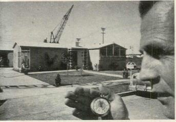
BUILDER HAL B. HAYES times erection of his prefabricated house which was assembled, furnished and landscaped in thirty-four minutes using mobile crane in background.
