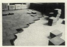
This concrete floor, insulated with PC Foamglas, prevents heat travel from the room below. A concrete wearing floor will cover the PC Foamglas.
