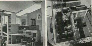
**MECHANICAL CORE**, of kitchen, bathroom and furnace closet swings into place in one unit. Plumbing fixtures are attached to walls in prefab assembly. Piping is built into walls. Center picture shows kitchen at end of living room. Picture on right shows unroofed unit with pipe air vent between kitchen and bath. Connections are made to water, gas and waste piping embedded in floor slab.
