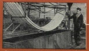
This is a hydraulic-plunger type of operation. In this model dead weights are eliminated, submerging is achieved by top side pressure. Tanks of this type are used for structural members and for fabricated pre-shaped stock, such as the Quanset arches pictured. Quantities of stock handled per immersion are comparatively small.
