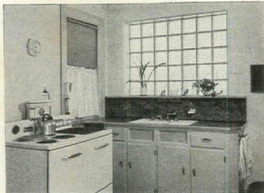
← **IN THE KITCHEN**—Panels of Insulux flood the work counters with natural daylight.
