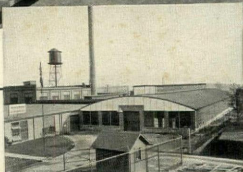
The completed plant and roof deck—incorporating 18,112 square feet of Cemesto.
