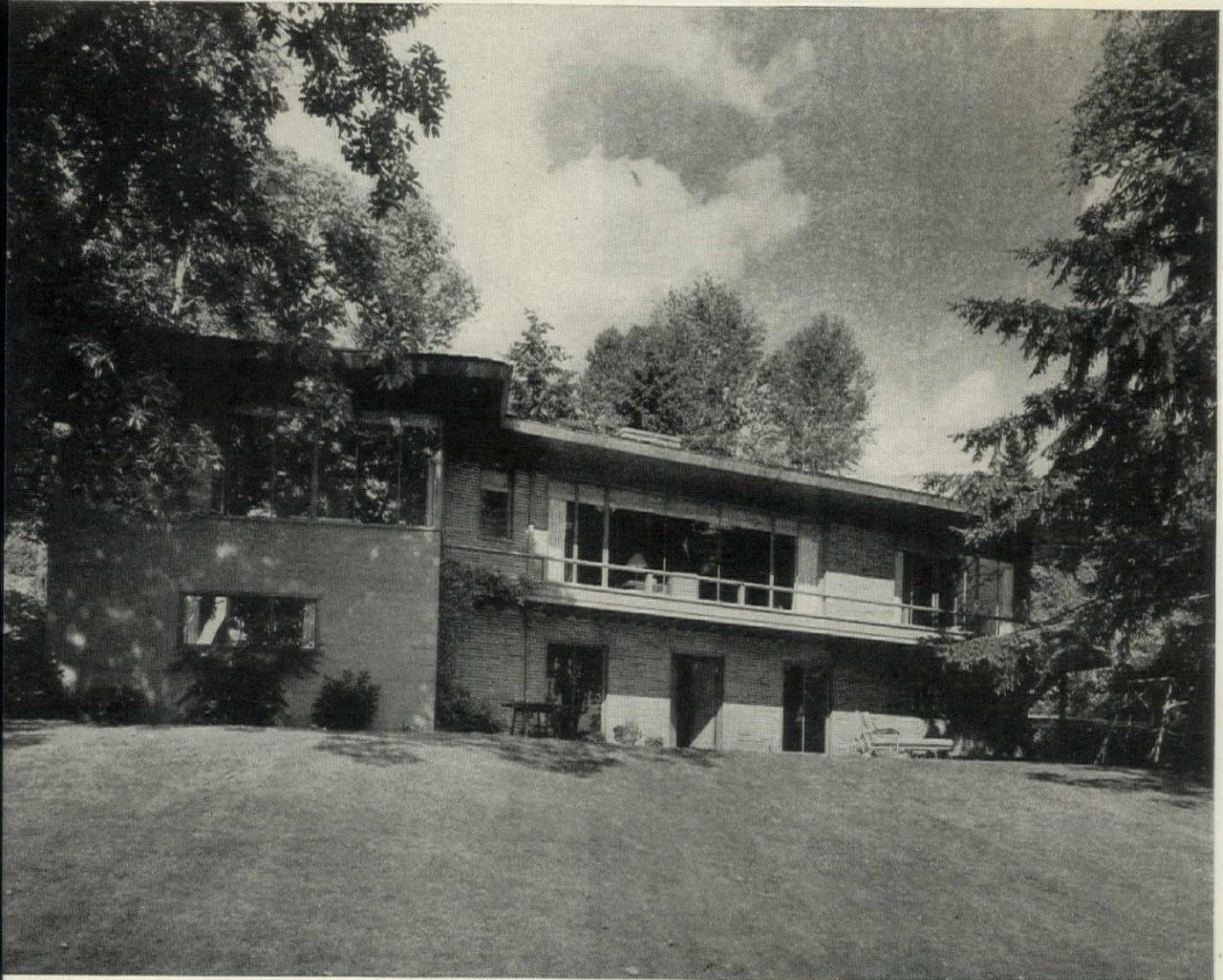
LIVING AND DINING SPACES ARE JOINED BY WIDE OPENING TO INCREASE VIEW OF LAKE STORY FACADE FACES LAKE, WITH LARGE WINDOWS SHIELDED BY ROOF OVERHANG AND CANTILEVERED BALCONY
