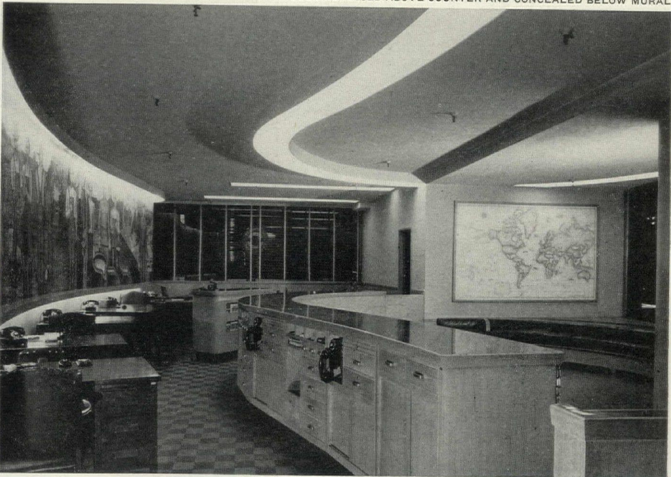
VIEW FROM SIDEWALK SHOWS CURVE OF TICKET COUNTER CONTINUED INTO SEATING FOR WAITING PASSENGERS WORK SPACES ARE LIGHTED BY COLD-CATHODE TUBES RECESSED ABOVE COUNTER AND CONCEALED BELOW MURAL
