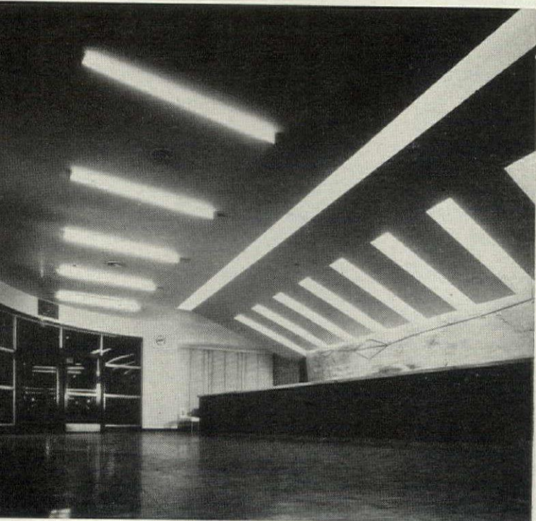
AREA IS LIGHTED BY EXPOSED TUBES, COUNTER BY COVES
