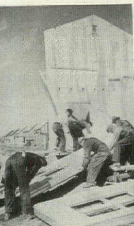
WALL-SIZE PANELS ARE DELIVERED FOR SITE ASSEMBLY BY THE OWNER
