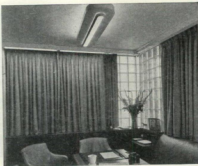
Study-type office or small conference room has lowered central fixture that provides both indirect general lighting and good working light on the desk itself.
