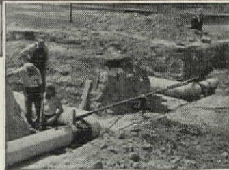
Ric-wil Prefabricated Expansion Loop "cold sprung" into position. Loops are fitted with drive couplers for easy assembly to straight runs.
