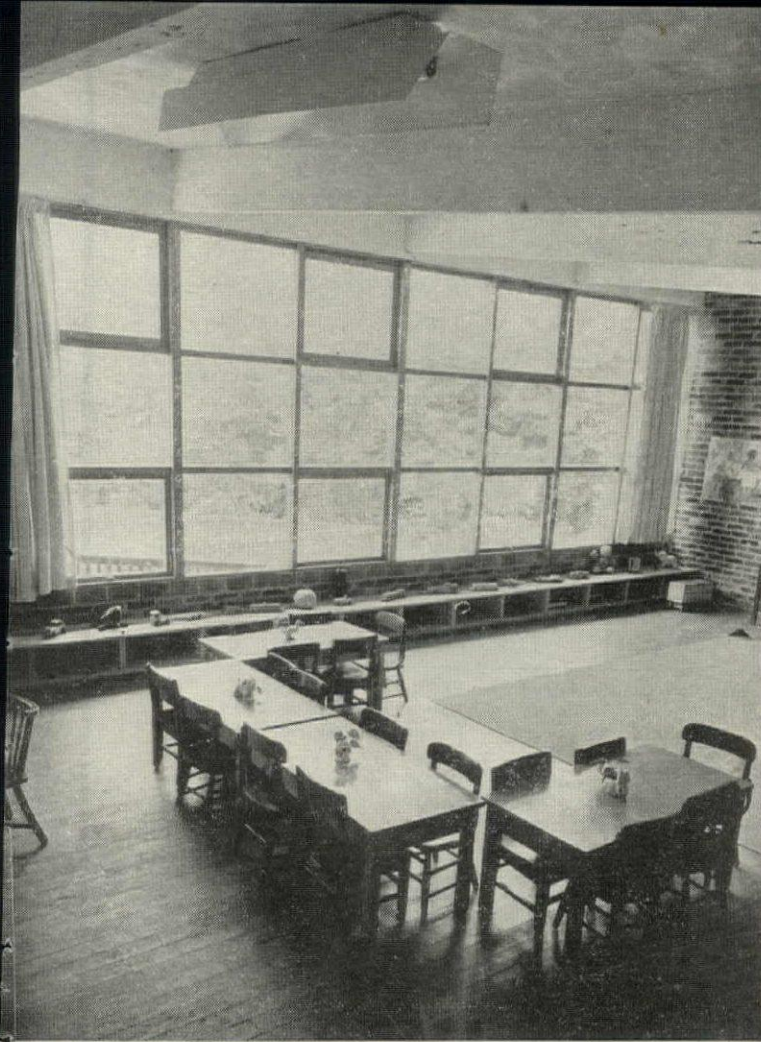
FIXED AND HINGED SASH NICELY VARY SCHOOL'S WINDOW GRID
