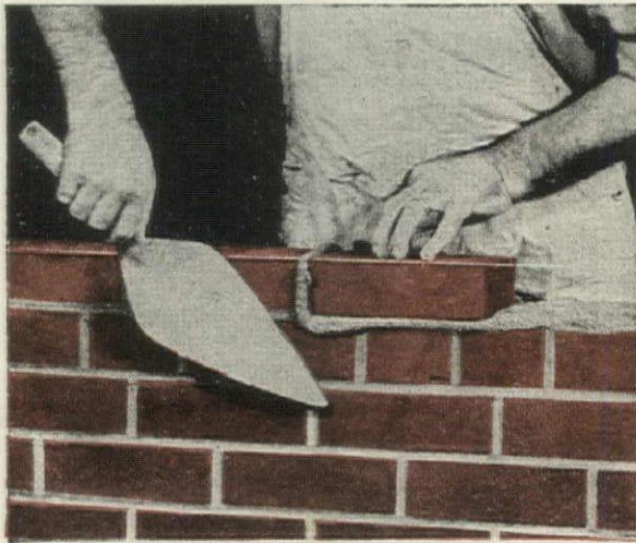
To make a good bond with the brick, mortar must be plastic, and stay plastic until the brick is bedded. The
