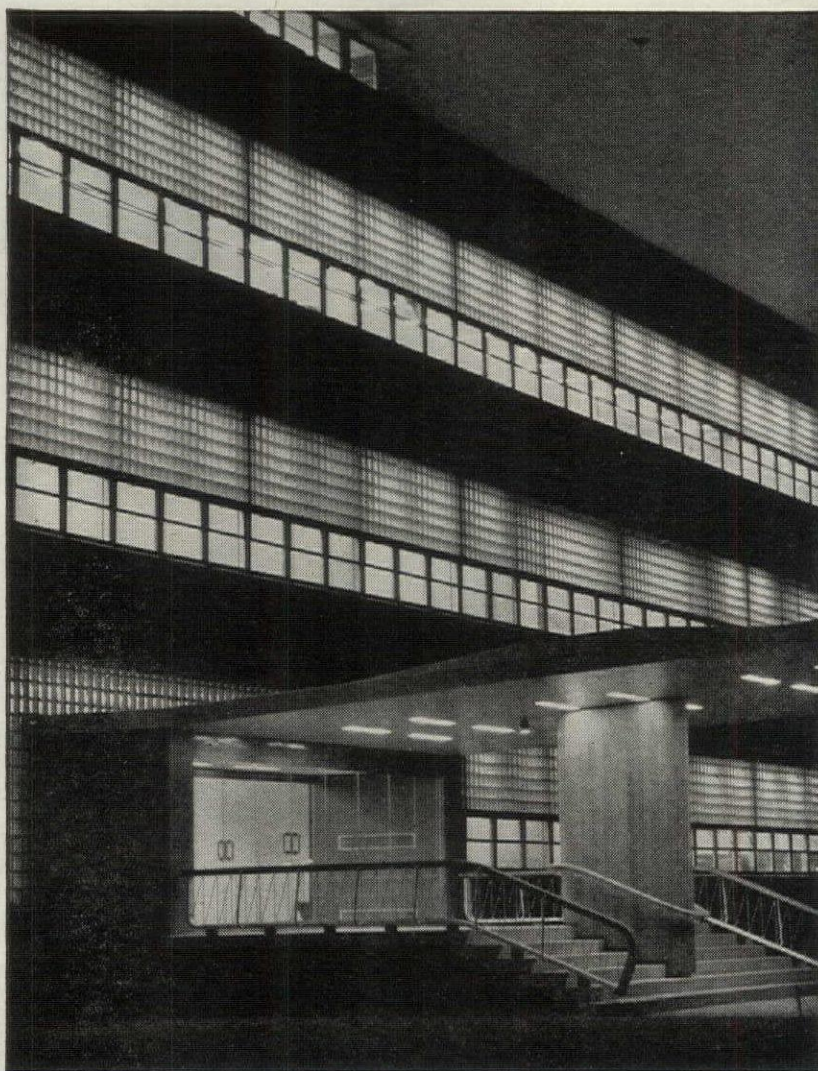
Night view of the Sperry Gyroscope Company's three-story administration building, designed by Nembhard N. Culin. This photograph shows dramatically how clear glass and prismatic glass block have been combined to distribute daylight and prevent glare.
