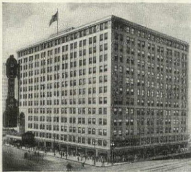
The Michigan building in Detroit which appreciates the advantages of Otis Elevator Modernization.
