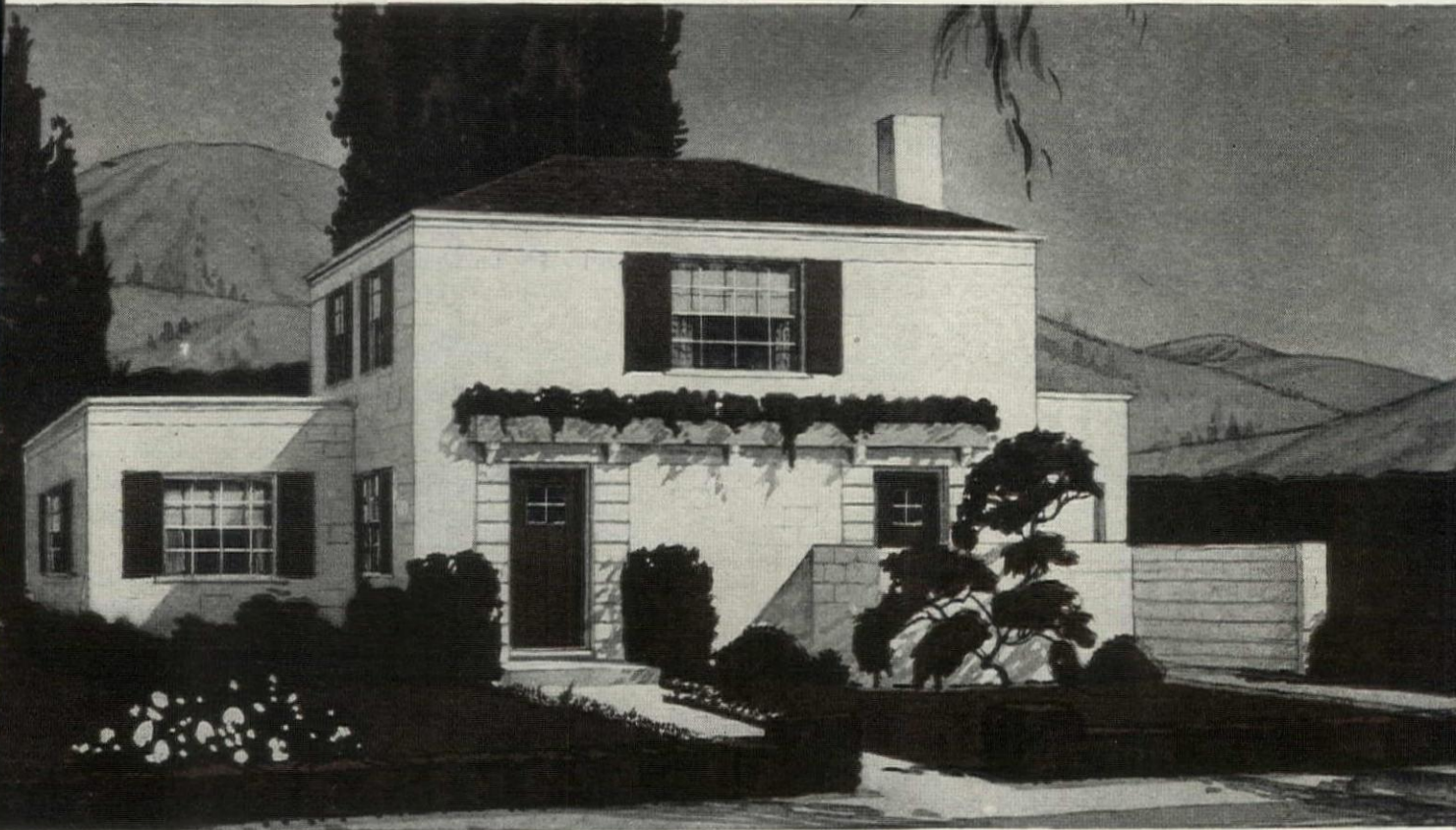
Designed for the Small Monthly House Club, Inc., by Chapman and Evans, Architects
