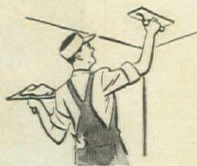
ACOUSTICAL PLASTER FINISH
