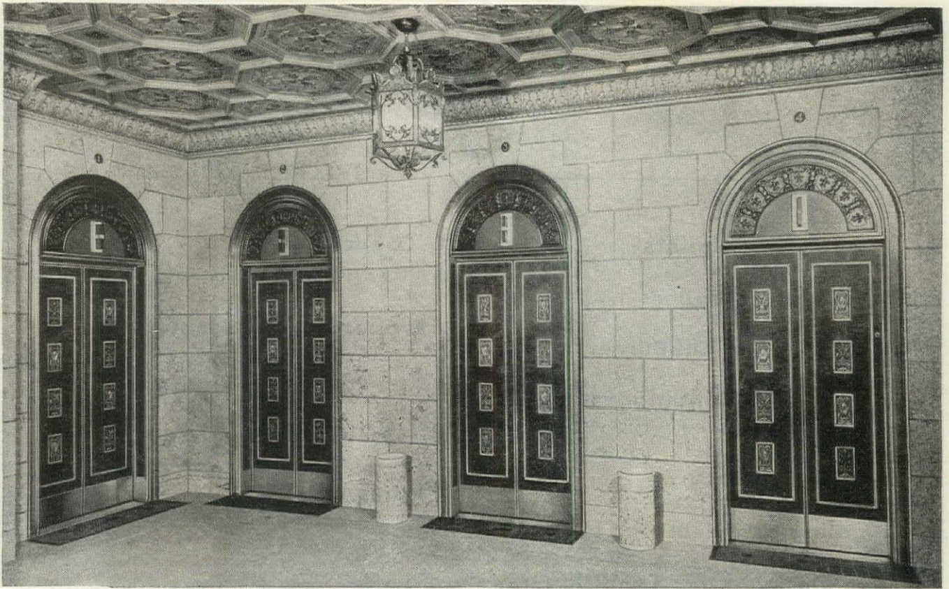
These beautifully designed, power-operated elevator doors replaced old-fashioned grille work.
