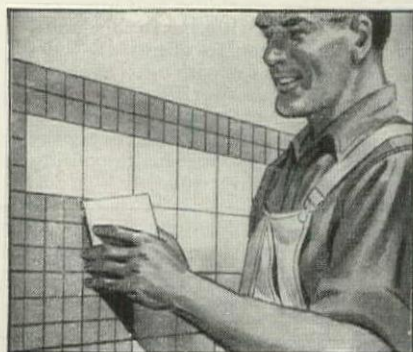
Formed edges of tile fit foundation sheet grooves which are designed to take all tile sizes.
