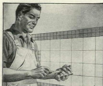
Waterproof adhesive applied to back of the tile insures life-time bond with foundation.
