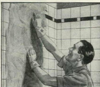
Rapid-setting waterproof white or colored cement grout fills the joints between the tiles.
