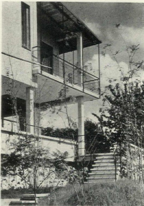
SIDE STEPS LEAD TO LIVING ROOM TERRACE
