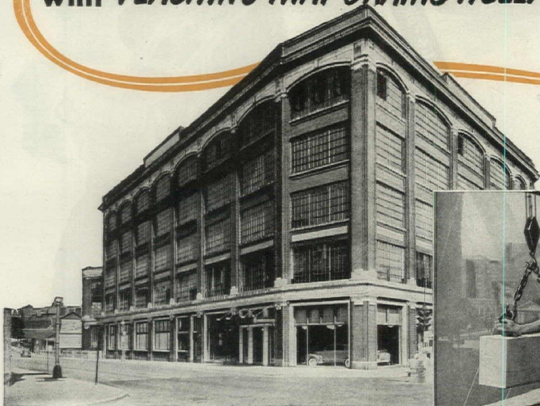
Automotive branch plant, in which 6,000 lb. of Anaconda Through-Wall Flashing were installed by Mandel Roofing Company, Pittsburgh, Pa.
