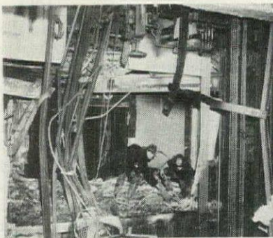
Wheels and undercarriage smashed through the 78th floor. One motor fell down elevator shaft.
