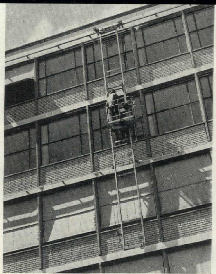
PERMANENT, MOBILE LADDER SIMPLIFIES WINDOW CLEANING
