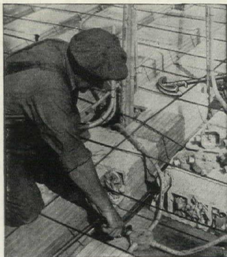
Simply spot the outlet and mount the box with necessary connectors already attached. Then run in the tubing at some later convenient time. On E.M.T. installations it is not necessary to turn the pipe—every connector is a union.
