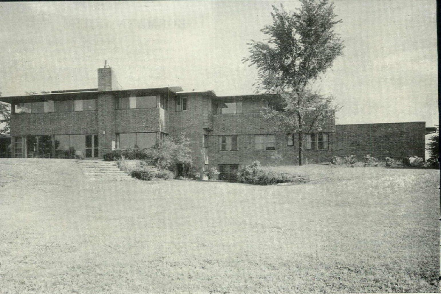
SOUTH ELEVATION REVEALS LAYOUT OF ENTIRE HOUSE. PROMINENT CHIMNEY SERVES SECOND FLOOR STUDY FIREPLACE
