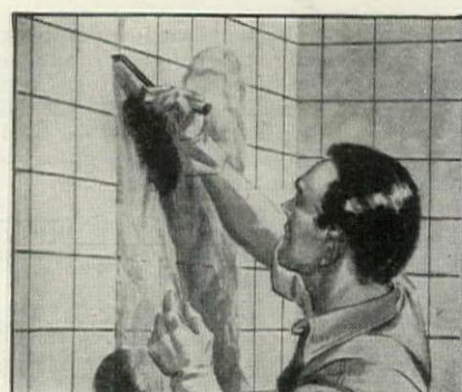
Squeegee removes excess grout; joints are pointed; tiles cleaned with sponge and fine steel wool.
