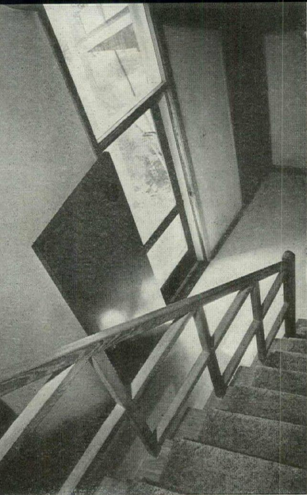
A SINGLE TRANSOM WINDOW LIGHTS STAIR HALL
