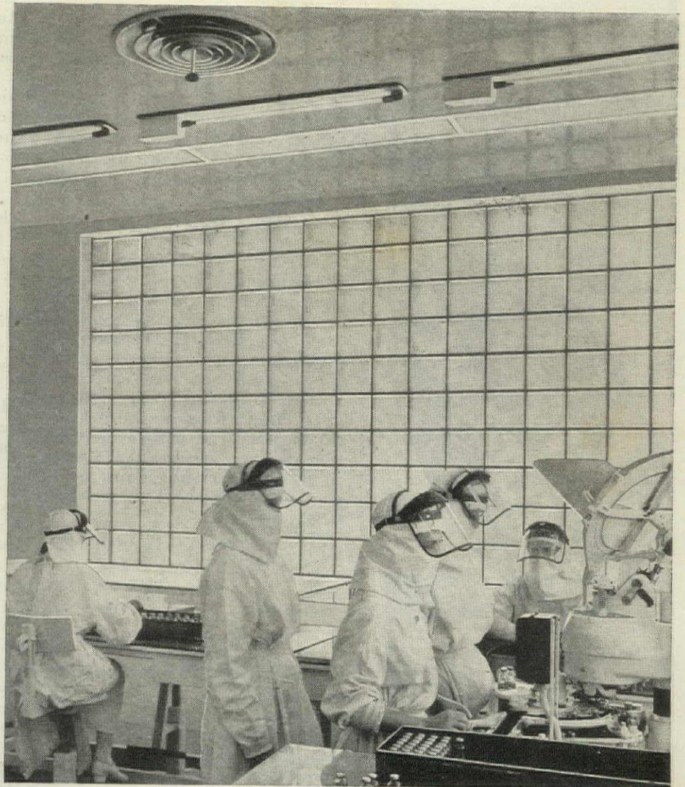
Interior New Penicillin Plant—Commercial Solvents Corporation, Terre Haute, Indiana
