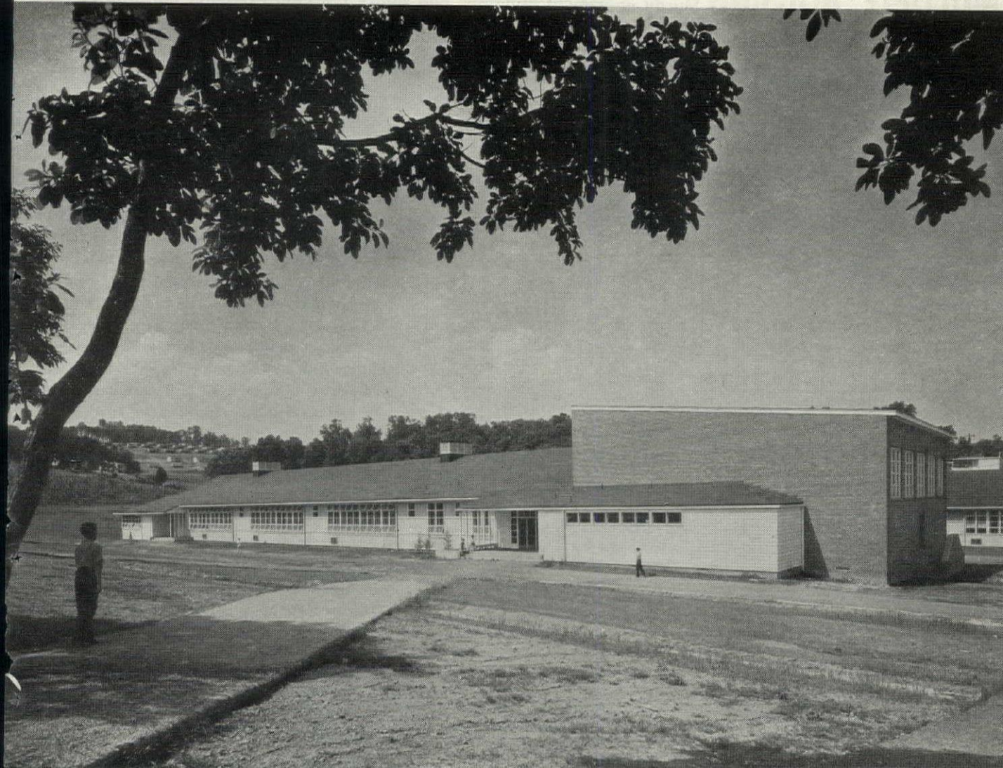
SCHOOL HAS CENTER ENTRANCE FLANKED BY CLASSROOM WING AND GYMNASIUM WITH SHOP EXTENSION AT REAR
