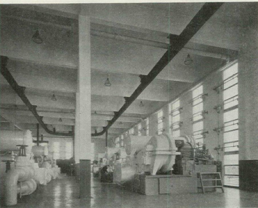
REFRIGERATING UNITS FOR AIR CONDITIONING ARE IN BOILER HOUSE
