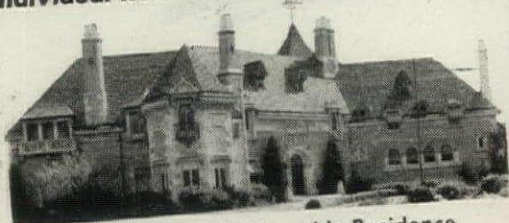
Mrs. Ella M. Weckbaugh's Residence Denver, Colorado Architect: The late J. B. Benedict
