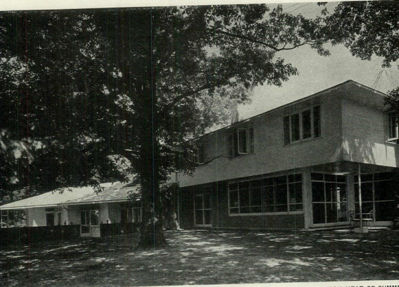
SOUTH FACADE HAS WIDE OVERHANGS AT ROOF AND SECOND FLOOR TO PROTECT HOUSE FROM HEAT OF SUMMER
