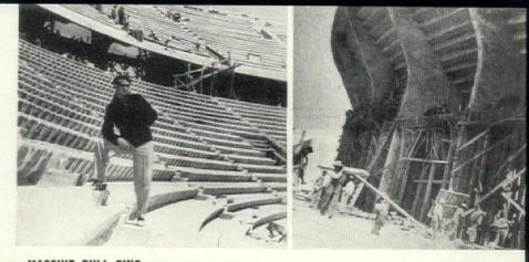
MASSIVE BULL RING shows off graceful lines of concrete construction. Complete scaffolding was erected, and concrete poured as continuous operation. Sculptor Albert Just (below, extreme left) is preparing bronze models of famous bullfighters to deck the seven gates. Promotor Simon (right) will build a University City next.
