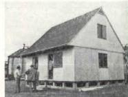
HOMEOLA, 20 ft. by 24 ft., is complete enclosed in a day by a small crew, no part weighs over 75 lbs.
