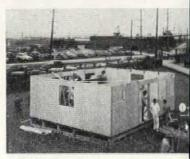
WALLS of first story in place, st joists to support second story a installed.
