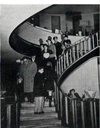
NARROW STAIRS seem to have been designed for a residence, not a busy terminal like LaGuardia. Picture shows unposed example of typical result during rush hours.
