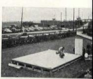
PREFINISHED floor panels, protect with paper, are installed over stujoists. Erection of outer wall begin
