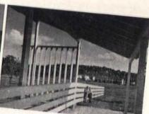
SIMPLEST POSSIBLE CONSTRUCTION WAS USED AT PINE FORD ACRES. INTERIOR OF NURSERY SHOWS EXPOSED STRUCTURAL MEMBERS. PLAY-GROUND OVERHANG IS MERELY EXTENDED ROOF SUPPORTED BY POSTS
