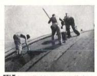
FELT is applied in mopping if slope is under 6 in. per ft.
