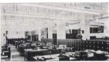
Chicago, III. Illumination at desk-level is 60 F.C. with 2.5 watts/sq. ft. FUTURLITERS are suspended from the 13'6'' ceiling to a 9'6'' mounting, and rows are on 7'0" spacings. Note the generous ceiling illumination. Engineered by Mr. G. A. Hall of the Guth Co.
