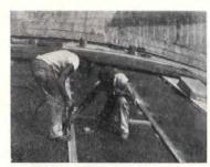
NAILING STRIPS are laid parallel to building's length.
