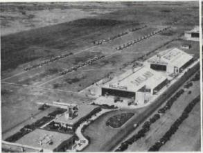
OAKLAND'S terminal cannot expand due to insufficient building area and crowding of adjacent hangars. Plan should provide for lateral additions to terminal.
