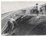
FELT is set in plastic cement if slope
