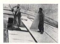
3 PLIES of insulating board are laid in asphalt mopping.
