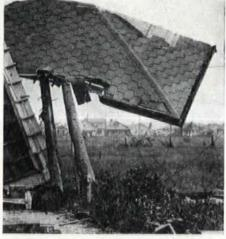
Roof deck blown completely off, but with practically every Cyclone shingle intact.
