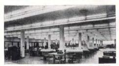
Houston, Tex. Using 2.9 watts/sq. ft., FUTUR-LITERS provide 54 F.C. The "45° Positioning" of drafting tables effectively reduces shadows. Ceil-ing-height is 10°", and fixture rows are 84" drafting tables effectively reduces shadows. Ceiling-height is 10'9", and fixture rows are 8'4" apart. Engineered by Mr. H. G. Hrivnatz of the Houston Lighting and Power Co.
