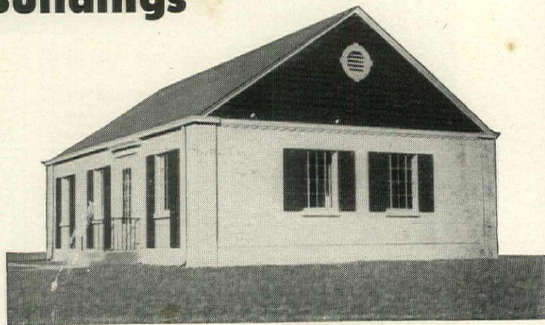
Five-room concrete house, built by Tilt-Up method.
