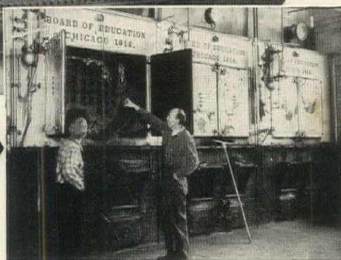
... replacing 3 tubular type boilers 60 x 18
