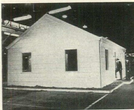
REYNOLDS ALUMINUM HOUSE experimental model is erected in factory at Louisville. Painted aluminum siding and conventional design makes aluminum house look just like frame cottage.
