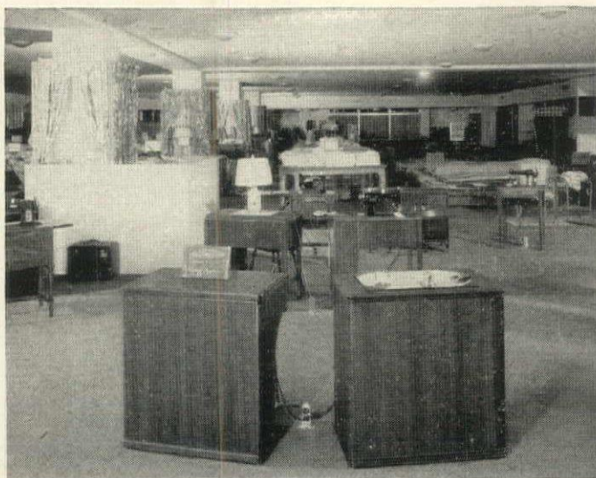
Above photograph is of a sales floor in a store with G-E Q-Floor Wiring. Note the many floor outlets in different parts of the room. Power is readily available for working models, etc.
