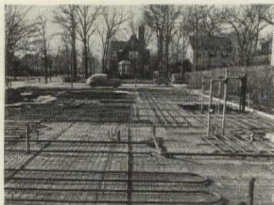
Typical floor installation of radiant pipe coils, just before pouring concrete.
