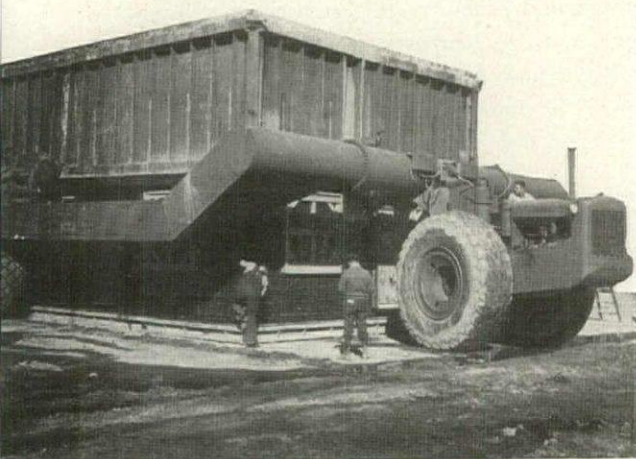
LE TOURNEAU MACHINE maneuvers on to building site on 12 ft., pneumatic-tired wheels, turns out a concrete house in 24 hours. Machine is as wide as a highway, is called Tournalayer.
