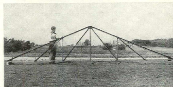
TWENTY-FIVE FOOT truss, weighing 293 lbs., was fabricated in 65 minutes. After completing ten trusses, workers could assemble truss faster than of comparable size could be bolted together. Detail shows apex of truss before painting.
