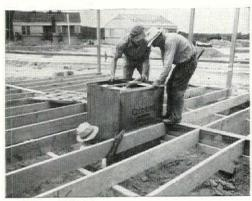
GRAVITY FLOOR FURNACES provide warm air heating in its simplest, most economical form and require no extra space. Picture shows a complete heating "system" being installed between floor joists in a basementless house. The heater is usually located in the living room floor where it heats other rooms by natural circulation of air. Manufacturer: Coleman Co., Wichita, Kans.
