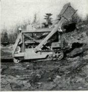
**EXCAVATING TOOLS.** left to right: a truck mounted augur drills holes for foundation piers; a "Caterpillar" tractor with "Trackson Traxcavator" lifts earth over wall of excavation; "Sargent Overhead" scoops up earth, swings it "over its head," dumps it into a truck.
