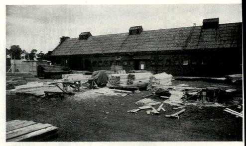
**CUTTING YARD AND SHOP.** Here Builders Place precut and store their framing members and assemble their shop-fabricated closets. The enclosed shop keeps labor busy during inclement weather, thus keeps construction of the project moving at all times.
