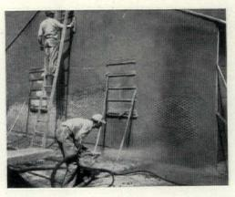
**GUNITE** reduced to simple terms, is simply stucco applied with an air gun. Compressed air and a thin mix of mortar are fed by separate hoses into a single nozzle. As a labor saving technique, its advantages are obvious. The photograph above shows the application of Gunite to the chicken wire lath of a small house, the windows of which have been temporarily masked to simplify the clean-up operation.
