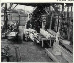
PRECUTTING of lumber in a shop or on the site saves time and eliminates waste of materials. Cutting is planned, and scraps are put to use. Scraps from hand-cutting on the site are usually considered useless and thrown away. Precutting is also more accurate.
