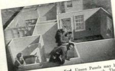
Easily, quickly applied. Upson Panels may be used either on steel or wood framework. They can be applied with regular Upson fasteners or by nailing and gluing.
