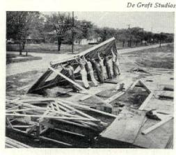
SITE FABRICATION is a compromise between shop assembly and conventional construction applicable to projects which are not large enough to warrant use of a big fabricating plant. Here, Builders Place (see p. 142) erect a wall which has been assembled on the floor.
