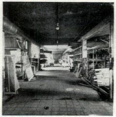
STORAGE RACKS inside the Place shop keep raw, precut and preassembled materials in order. Materials are stored until required on the job, thus reducing weather damage and loss. Windows and screens are stored to the left; trim, to the right.
