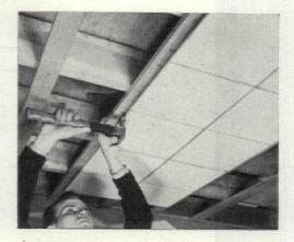
SMALL PANELS of composition board used as interior finish may be laid with joints accentuated. The resultant tile-like pattern overcomes the public's dislike of the difficultto-conceal joints which occur ungeometrically in large-panel wall finishes. The picture shows the ceiling installation of Wood Conversion Co.'s "NU-Wood" tiles with special clips which make concealed nailing possible. Available in various fade-proof colors, such prefinished materials eliminate the need for interior painting.
