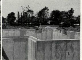
STEEL FRAMEWORK REINFORCES PLYWOOD FORMING PANELS, REDUCES SHORING AND PRODUCES A TRUE, SMOOTH WALL OF CONCRETE
