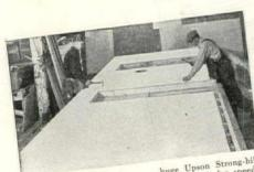
Full-wall Panels . . . huge Upson Strong-hilt Panels are 8' high and room-length for speedy factory assembly. Openings cut out quickly with power saw. No ugly nail holes or taped joints with true Upson full-wall construction.
