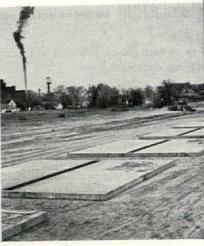
FINISHED SLABS line the street of the Place project. Rectangular slab in foreground is for a three-bedroom house; L-shaped slabs further down the line will accommodate two-bedroom units. Houses 30 ft. wide on lots averaging 40 ft. in width leave only about 10 ft. between adjacent buildings.
