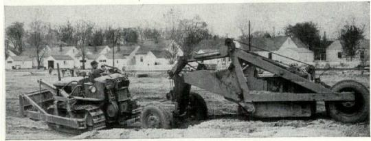
BULL DOZER AND SCRAPER were the biggest tools rented by Place and Co. to assist in the construction of their 180 South Bend house (p. 142). Main jobs: grading and back-filling.
