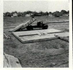
**DELIVERY** of materials is timed to coincide with their need. Here a truckload of precut framing members and plywood panels is dumped at a completed floor slab. Cable in foreground supplies power to electric tools used on the site.
