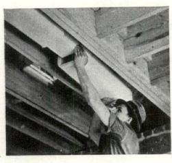
ASBESTOS DUCTS fit between floor framing members. Lightweight sections are put together by means of slip joints which are sealed to prevent escape of air. Made entirely of asbestos, the sections may be cut with an ordinary saw. Manufacturer: Philip Carey Mfg. Co., Cincinnati, Ohio.
