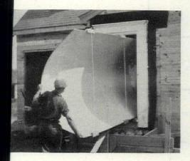
ARGE SHEETS of plaster, fiber and other omposition boards offer obvious economies in nterior finish. For instance, the large sheet f Upson Co. fiber board bent to go through he front door (above) will finish one entire vall of an average size room having an 8 ft. eiling. Moreover, the panel is factory-primed, will therefore require only one coat of paint. Dry wall construction of any type keeps moisure out of the house and thus saves time in he application of interior finish.
