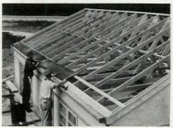
NAILED TRUSSES accomplish the same purposes as those described on the left, but involve more labor. In these houses designed by the Pierce Foundation for the Glen Martin plant in Baltimore, both the upper and lower chords of the trusses are 2 by 4's. Shear resistance of nailing was augmented by notching the upper chords into the lower chords.
