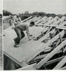
ROOF SHEATHING is ½ in. plywood. It will be finished with mineral surfaced asphalt shingles. Trusses span the entire main element of house, make structural partitions unnecessary. Ceilings are blanketed with cotton insulation. Attic space is ventilated by factory-made metal louvers at either end.
