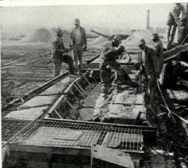
CONCRETE POURED INTO MOLDS AT CAST
