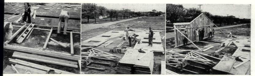
AYOUT PLATES are fabricated of 1 by 4's with leces of waterproof plywood carefully spaced to orm notches into which studs are dropped for erfect alignment. Serving the purpose of a refabricator's jigtable, these layout plates are arried from house to house. Slab has been nopped with asphalt and will be covered with leepers and prefinished oak flooring.
