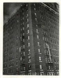
FIREPROOF steel-and-concrete exterior of structure was completely undamaged by fire in which 61 guests died. Old-fashioned exterior fire-escape proved completely inadequate. Many guests tried to escape by tying bed sheets together; most could not find fire escape.
