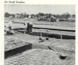
SLAB foundation for the Place house (page 142) requires a minimum of forming lumber. Pipes are laid in the tamped earth base; shallow trenches are dug for footings; reinforcing mesh and rods are positioned; then the concrete is poured inside perimeter forms. Slab forms are prefabricated from 2 in. by 12 in. planks connected with large strap hinges from
