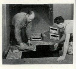
DIRECT ADHESION TILE is mounted on a hair-thin plastic sheet and is applied with an adhesive to any true surface-wood or concrete floors and dry-built walls. This new plastic development makes for quicker and lighter installations. Cement is needed only for grouting. No opaque paper pasted to the face of the tile hinders the alignment of sheets, which measure 12 in. by 24 in. Manufacturer: U. S. Quarry Tile Co., New York City.
