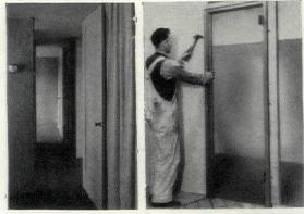
INTERIOR DOORS which reach the ceiling (left above) save materials and tedious lintel construction. Factory fabricated steel door frames save time and money and assure a true door opening. Picture (right, above) shows installation of a steel frame manufactured by New York's Aetna Steel Products Corp. For a close-up of a similar installation in the Place project, by Richmond (Va.) Fireproof Door Co., see p. 142.
