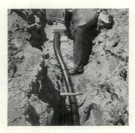
SEWER PIPES of clay are hard to get. Comparable in initial cost but more readily available and much easier to lay is the pipe produced by Fibre Conduit Co. of Orangeburg, N. Y., pictured above. Available in lengths up to 8 ft. the pipe is tapered at either end and Joined with a friction sleeve which requires no cementing. Perforated pipe is available for foundation drains and septic tank filter drains. Similar bituminized-fiber pipe is manufactured by Brown Co., New York City.
