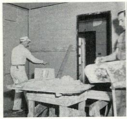
PARTITIONS are made of solid plaster 2 in. thick. Horizontal brace holds large sheets of gypsum lath rigid while plaster scratch coat is being applied to both sides. Partition above butts against an exterior wall which is lathed with gypsum sheets ready for plastering. For details of solid plaster partitions see page 120.
