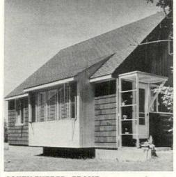
GANTILEVERED FRAME increases the size of the house without increasing the volume of excavation and the perimeter of the foundation. This economical practice may be carried much further than did Architect Samuel Glaser in the small house pictured above in which the living room extends beyond the foundation. In two-story houses, the second floor may be expanded to produce premium second-floor space if cantilevered beyond the first floor.
