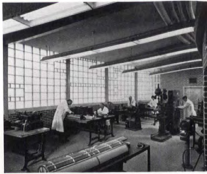
EXPOSED CAVITY BRICK WALLS DELICATE WELDED BENTS MAKE UP THE HANDSOME FRAME GLASSBLOCK PANELS HAVE INTEGRAL PATTERN
