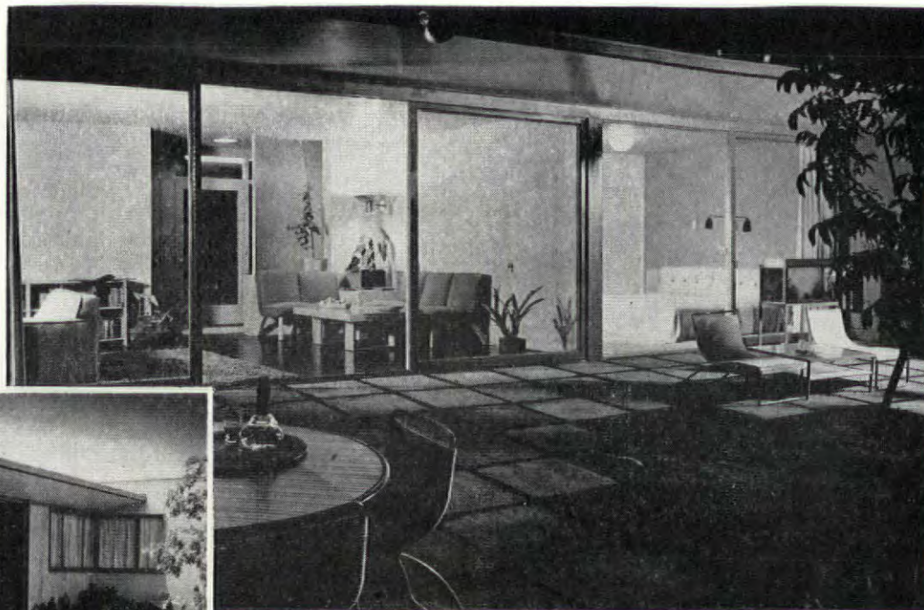
COMPLETED LAST MONTH is Case Study House No. 11, designed by architect J. R. Davidson. Smallest of Arts and Architecture-sponsored plans, No. 11 is a four-room, one-story house scaled to veteran requirements. Built on radiant-heated concrete slab, it is walled with beige-finished stucco and room-high plate-glass.
