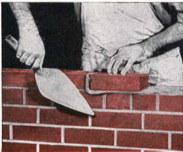
To make a good bond with the brick, mortar must be plastic, and stay plastic until the brick is bedded. The
