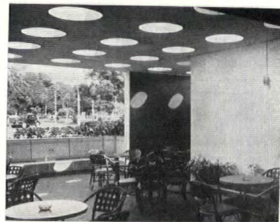
SPANISH PATIO , opening off bar, has tile floor, plaster walls and reinforced concrete slat roof, pierced by circular holes for shade and ventilation.
