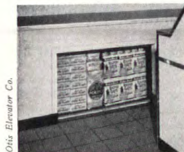
DUMBWAITERS are essential where entire layout is not on one floor. Illustrated model is suitable for movement of supplies or prepared foods from one floor to another. Other types employ regularly spaced lifts on continuously rotating belt.
