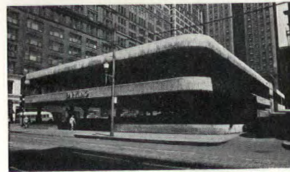
OPEN-WALL, MULTI-DECK garages are inexpensive to build, easy to maintain, are finding growing favor with department stores like Kaufmann's, Pittsburgh, which built building above.
