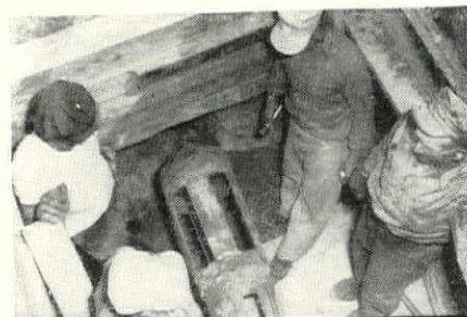
(Left) Normal traffic was maintained on this busy downtown street while Ric-wil units were installed under pavement. Units were jacked through from building basements and joined to utility's steam main at manhole in center of street. (Right) Close-up of manhole showing auger crew and tool for drilling under pavement.
