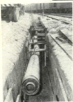
21 ft. Ric-wil Prefabricated Insulated Pipe unit lowered into trench alongside tracks at RR passenger station without interrupting rail traffic.
