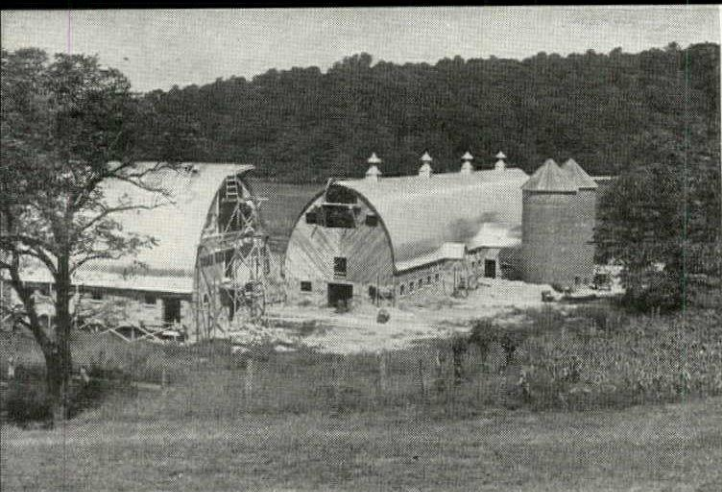
ALUMINUM ROOFING by Reynolds landmarks farm buildings. Sheeting, rolled from airplane scrap, is in galvanized-steel price range. V-crimp style roofing (at right) provides good bearing surface.
