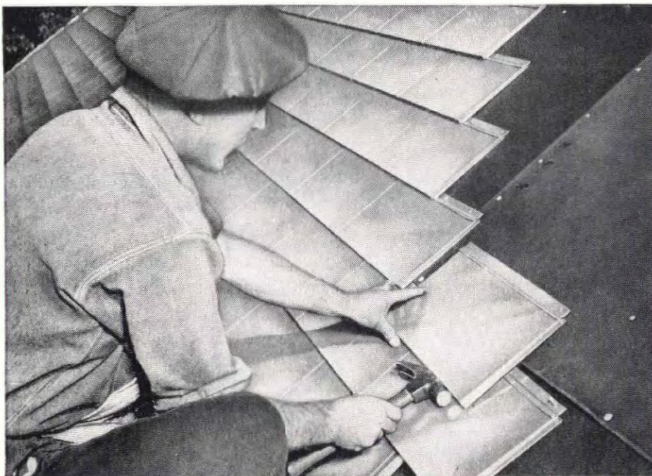
Reynolds Lifetime Aluminum Shingles being applied on a fine home in Kentucky. Note the attractive shadow line, the ease of application and simplicity of design . . . for a lifetime roof.
