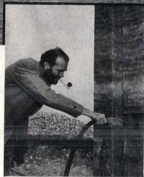
DESIGNER BOGGS plays a hose on a new earth wall to demonstrate its surprising resistance to weathering. Soil from the excavation (left above) was used to build the house at right.
