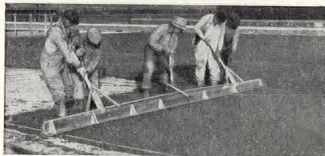
• Screeding Zonolite Insulating Concrete roof fill over concrete slab. Easily formed into saddles and cants for proper drainage.
