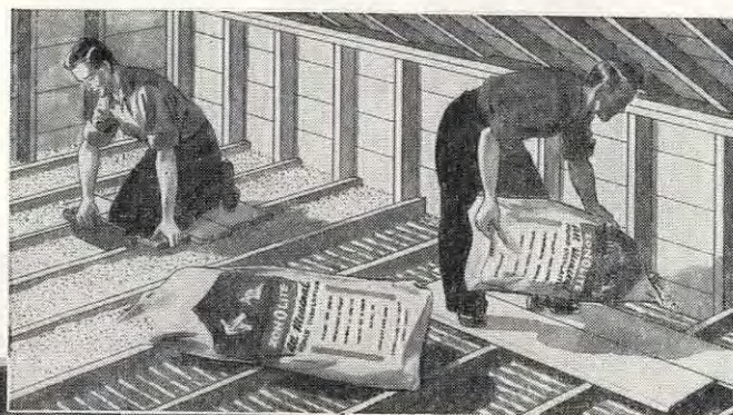
• Zonolite Granular Fill easily installed in attics and sidewalls—new work or remodeling. No gloves or masks needed.
