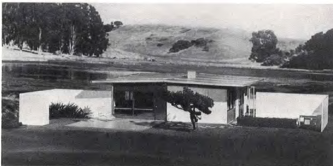
FIRST AIRCRAFT PREFAB to be unveiled is this model of aluminum house slated for manufacture by Consolidated Vultee Aircraft. Convair house has been approved for future contract. Cost, $7,000-8,000.
