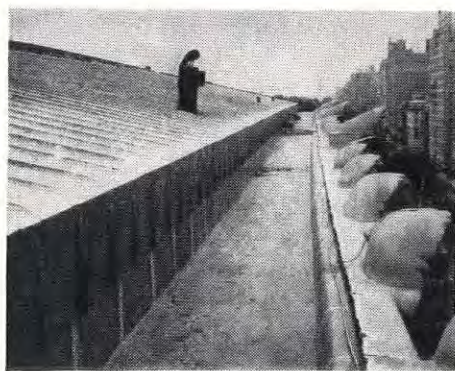
VIEW OF MONEL GUTTER and section of standing seam roofing and flashing installed in 1936.
