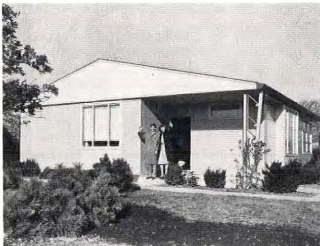
LUSTRON HOUSE , most headlined recent prefab, is trim, up-to-date design. Made entirely of non-glossy enameled steel, inside and outside surfaces are permanent, washable. Cost, around, $7,000.
