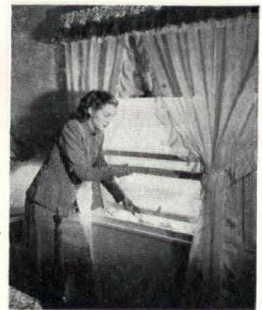
WINDOW is awning type; lower two-thirds swing out; inside screen slides up.
