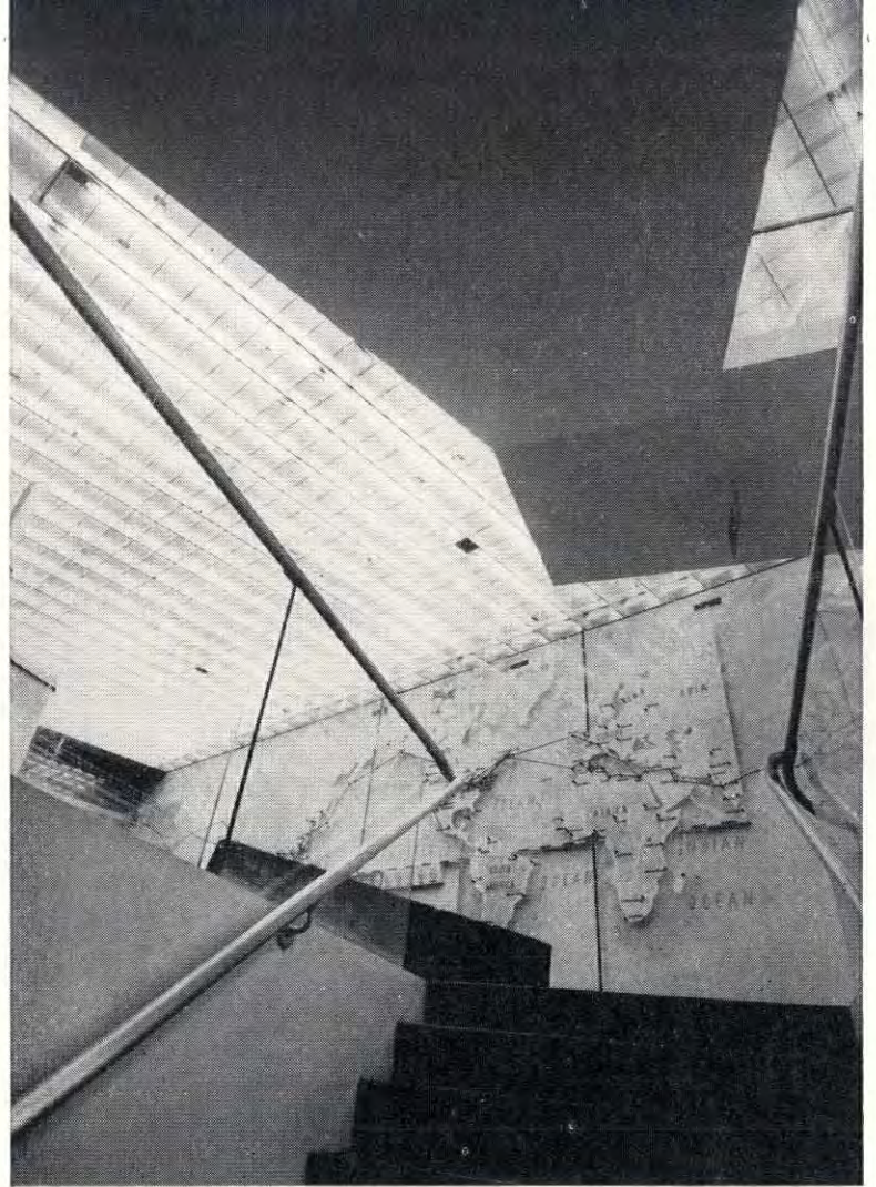
STAIR HAS HERCULITE RAILING TOPPED BY ALUMINUM HANDRAIL
