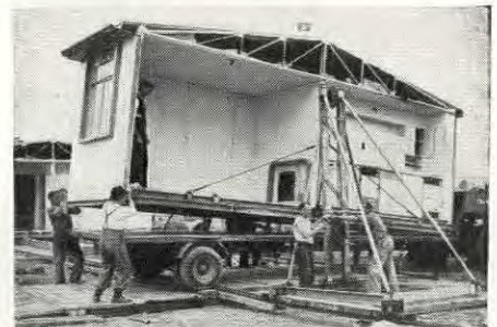
UTILITY CORE is trucked to site (above) and lowered onto its foundation by crane (below).
