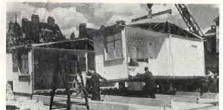
UTILITY CORE is trucked to site (above) and lowered onto its foundation by crane (below).
