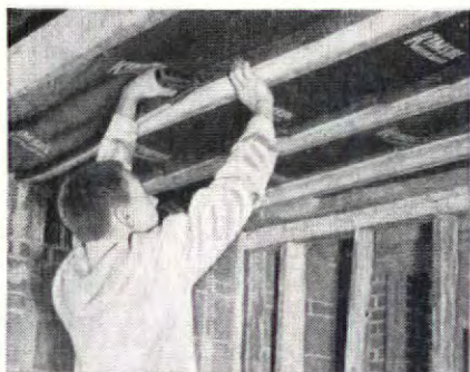
Installing light, flexible KIMSUL* in a CAPITOL PROPERTIES, INC. home. It is easy—just cut KIMSUL to desired length, expand it, and staple to ceiling joists.
