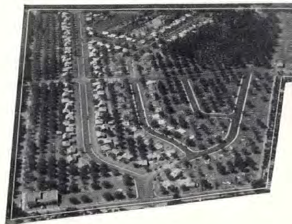
IN A SAN JOSE ORCHARD are 173 houses under construction, room for 627 more. These houses are completely site-fabricated but are otherwise the same as the factory-made units. Note staggered building line.
