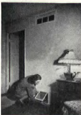
GRAVITY HEATER of vertical design is gas-fired, requires less space than an average closet. Cold air vent at floor and warm air ejection at ceiling create forced air action.
