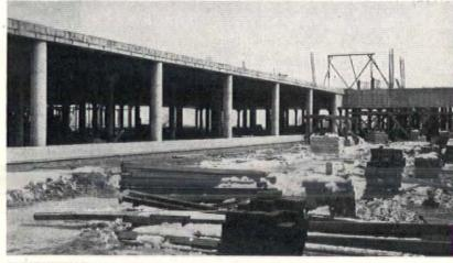
**CONSTRUCTION** throughout main work areas (above) is reinforced concrete with mushroom columns spaced 25 ft. on centers. Only exceptions are retail shop, garage, cafeteria and boiler house of structural steel to permit large unobstructed spans.
