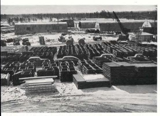
WALLS of welded steel are shop-fabricated, field-finished.
