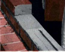
Then the excess mortar will fill the furrow and insure full bed joints.
