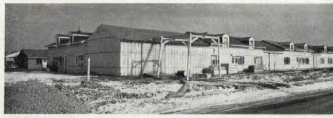
FABRICATING SHOP in center of site is comprised of five house shells, which will ultimately finished for sale, therefore represents a minimum plant investment. Panels are stored in near e of 5,400 sq. ft. shop, moved out by overhead conveyor for truck delivery to building sites.
