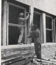
PAIR OF WINDOWS (left) is installed between outside columns. Like columns, gap between is covered with crimped, prefabricated, stainless steel facing.
