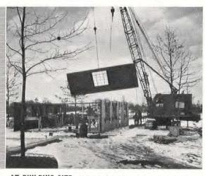
AT BUILDING SITE wall panels are swung into position, bolted to foundation and temporarily wired together. First two walls are held by temporary rigging. Heaviest wall: 1,200 lbs. Scaffolding is for later use of welders.
