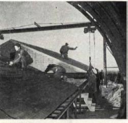
THIRD STAGE of assembly involves application of asphalt shingles over building paper. Prior stages (not shown) include 1) welding trusses and braces into rigid frame, 2) nailing wood sheathing to trusses, stucco lath to gable ends. Completed roof is lifted while truck backs under.
