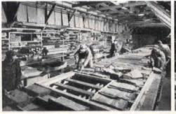
ABRICATION of panels is facilitated by storage of precut members in umbered pigeonholes opposite point of use. Sets of colored tabs on g tables align members for framing of any type panel on any table.
