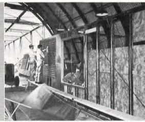
VERTICAL RACK holds panels while paper and lath are nailed to inside (near) face of studs and glass insulation board and paper-backed stucco lath are affixed to outside (far) face with the aid of welding gun.
