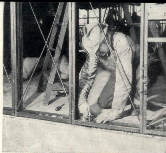
PREFABRICATED FRAME IS BOLTED TO CONCRETE SLAB
