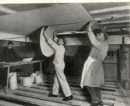
IDEAL FOR REMODELING , Crittall's heating element comes in 100 ft. strips, may be cut every 2 ft., has 2 in. selvage for stapling to joists.
