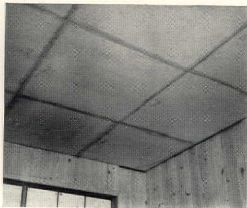
NAILED DIRECTLY TO RAFTERS , panels are connected by electricians from above, then covered with 8 in. insulation fill. "Blank" panels are used in those portions of the ceiling where no heating is required.
