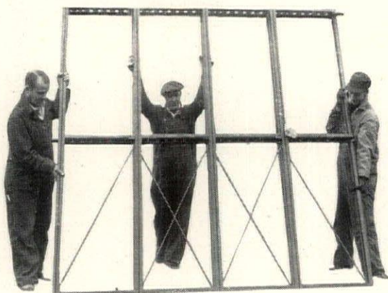
STEEL FRAME ASSEMBLIES , factory welded, are easily handled by three men. Typical house requires 20 wall sections of 11 different types, six partition panels, several storage partitions and ten trusses.
