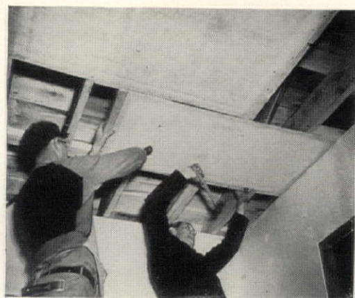
JOINTS TAPED , panels are ready for finish. Paper or paint may be either applied directly to fabric surface or on top of very thin coat of finish plaster.
