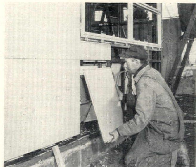
EXTERIOR PANS INTERLOCK, ARE SCREWED TO FRAME
