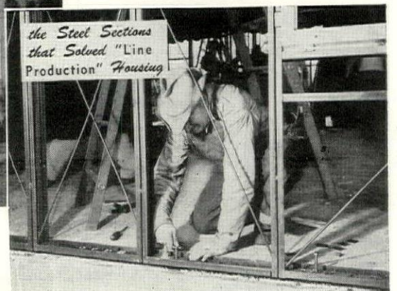
No. 3 AS STUDS AND ROOF TRUSSES for prefabricated houses as used in the LUSTRON HOUSE. Porcelain enameled plates are attached to Macomber V Studs with metal screws. At right, bolting Macomber V Stud panels to LUSTRON HOUSE foundation.
