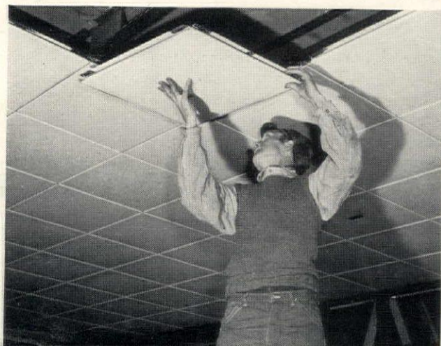
CEILING PANS FORM THE RADIANT HEATING SURFACE
