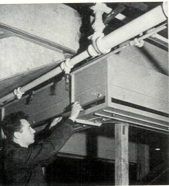
PROPOSED INSTALLATION of new control system around moving stairway in Hartford, Conn. store (above) contains same elements as in test unit (left): however, they are concealed in new soffit.
