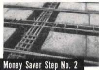
In this photograph, the reinforcing bars are installed as detailed by Ceco, in proper relation to the erected steelforms. Now the job is ready for placement of the temperature mesh in the top slab. This mesh reinforcement is also supplied by Ceco.
