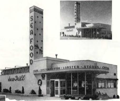
Inside walls are of Interior-type Douglas fir plywood. Ceiling, also of plywood, is covered with sound-absorption blocks. Outside walls, including the pylon, are Exterior-type plywood, as are two walk-in refrigerator units for fish and meat storage.
