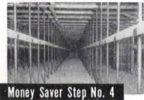
Underneath the concrete joists, Meyer adjustable steel shores support the open wood centering. Forming the floor construction above are adjustable-type steelforms nailed to the centering. Also available are flange-type steelforms, used when plastered ceilings are to be installed.
