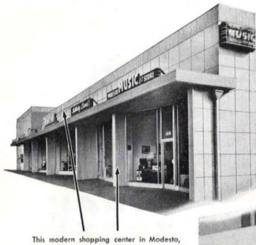
This modern shopping center in Modesto, California, makes use of Zourite as a facing for the walls which separate the stores and as a decorative covering for the cornice. On Dean's Drug Store in Niles, Michigan, Zourite has been applied vertically to the exterior wall and horizontally to the sign area above the projecting ceiling ledge.
