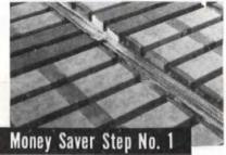
Meyer steelforms completely erected on open wood centering, ready for placement of reinforcing steel and concrete. Note column spirals awaiting installation in columns. Ceco engineers lay out and supervise the complete installation of steelforms on open wood centering.
