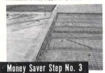
Here the mesh, also known as welded wire fabric, has been placed in correct position and the pouring of concrete for the top slab has commenced. In Cecorected jobs such as this, the design is carefully engineered to assure proper reinforcement throughout the structure.
