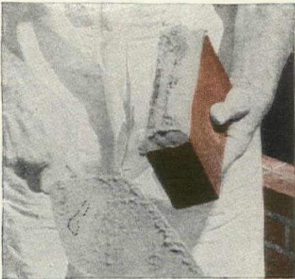
Mortar should be spread over the entire side of the header brick before it is placed on the wall.
