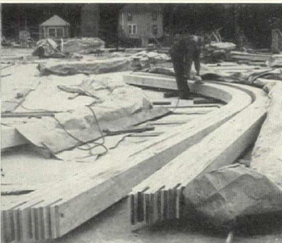
**SANDING** of completed lower chords was done with a portable sanding machine. Chords were then placed on jig tables for final assembly with rectilinear members to complete the arch.
