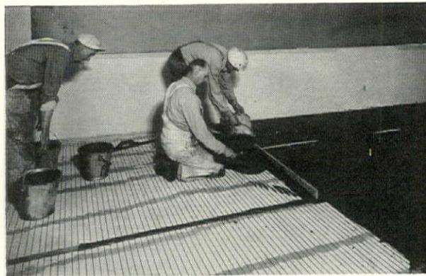
3. When floor has set properly, finish coat is polished with ordinary sander. Photo at right shows five sizes in which bark "aggregate" is produced.
