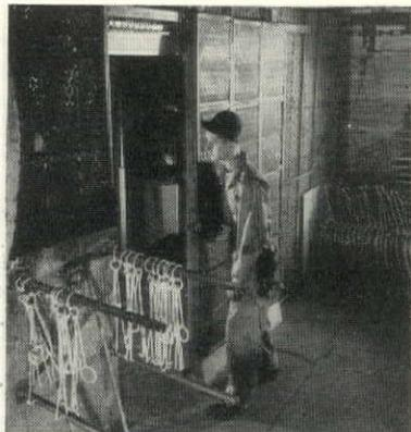
DUST-STOPS mounted on this sliding door provide filtered protection for sensitive electrical controls.
