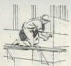
Big, weatherproofed panels of Gold Bond Storm Sealed Gypsum Sheathing add structural strength and built-in fire protection. Costs less than old-style sheathing.
