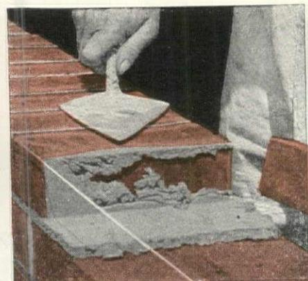
Slushing will not fill the voids.
