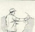
Over the plaster, goes a coat of Gold Bond Finish Lime. This is the smooth white finish that you see in a new house before the wallpaper or paint is applied.
