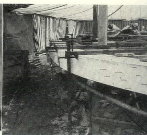
**ADHESIVE** was spread on inside of each successive plank. Then, working from one end of template plank was bent into place, pre-set nails driven home. Another ply had been added.
