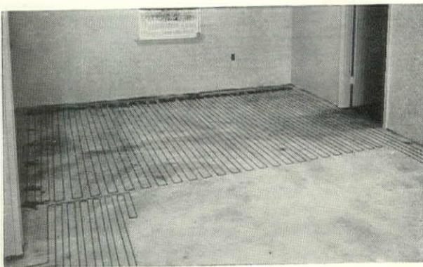
1. After scratch coat of bark and magnesite is poured and screeded, resistance coils are laid out and tacked in place.
