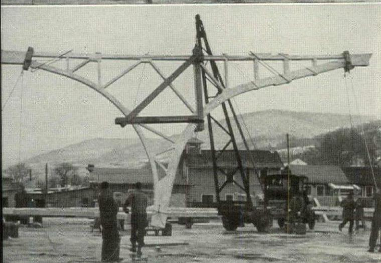
Foot of arch is fixed in steel hinge anchored to concrete foundation.
