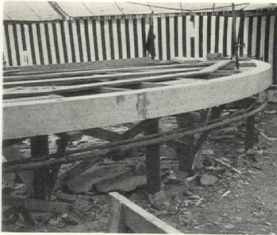
**STEAM-HEATED TEMPLATES** sped site fabrication of hinged arches during cold weather. Using a waterproof resin and engineered nailing pattern, lower chord of arches was built up to 15 plys.
