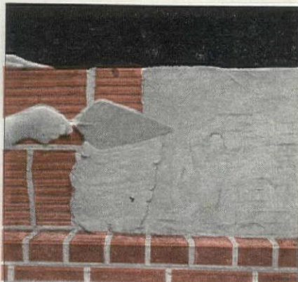
Or if the back-up units are laid first, the front of the back-up units should be plastered in the same way.
