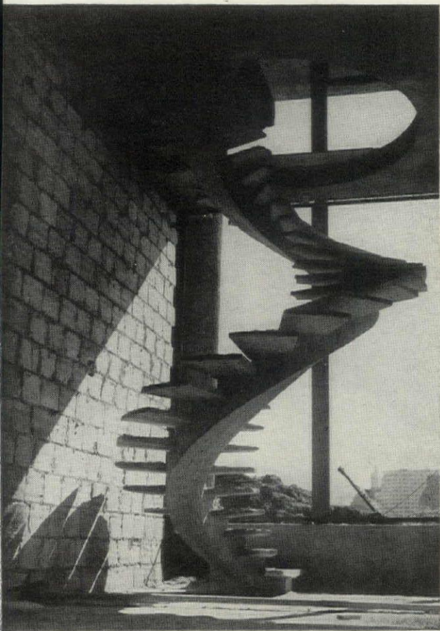
SCULPTURE in reinforced concrete, these stairs connect the telegraph booth (near main entry) with a second floor office.
