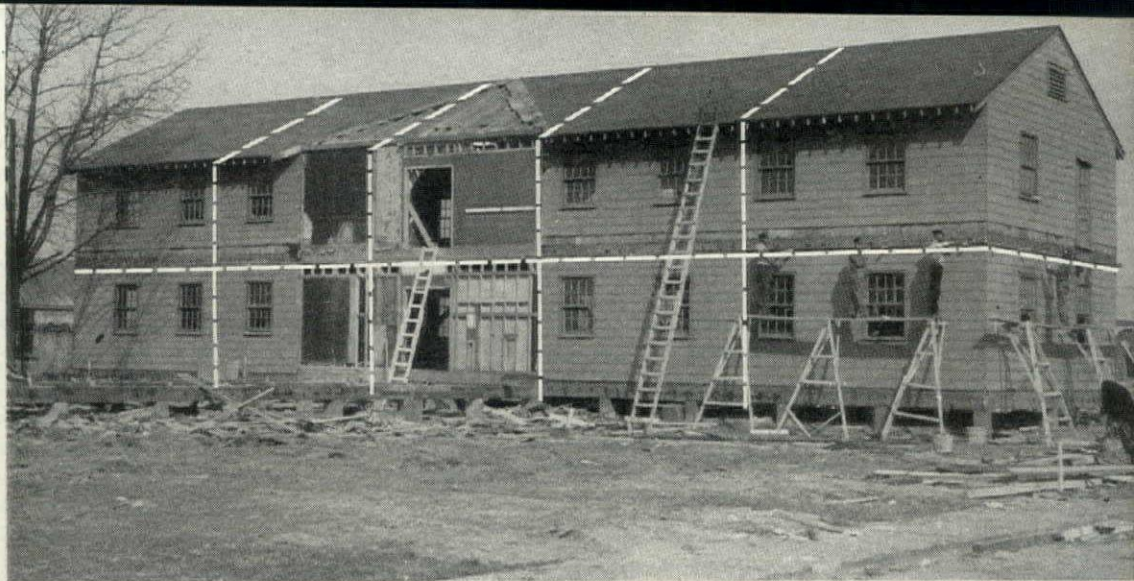
TEN H-SHAPED BARRACKS were sawed into 181 houses. Each side wing was cut five times; thus five 28 x 20 ft. sections were cut from each floor. First-floor sections had to be roofed. Roofing came from 28 x 112 ft. central wing—cross bar of H. This also supplied end walls.
