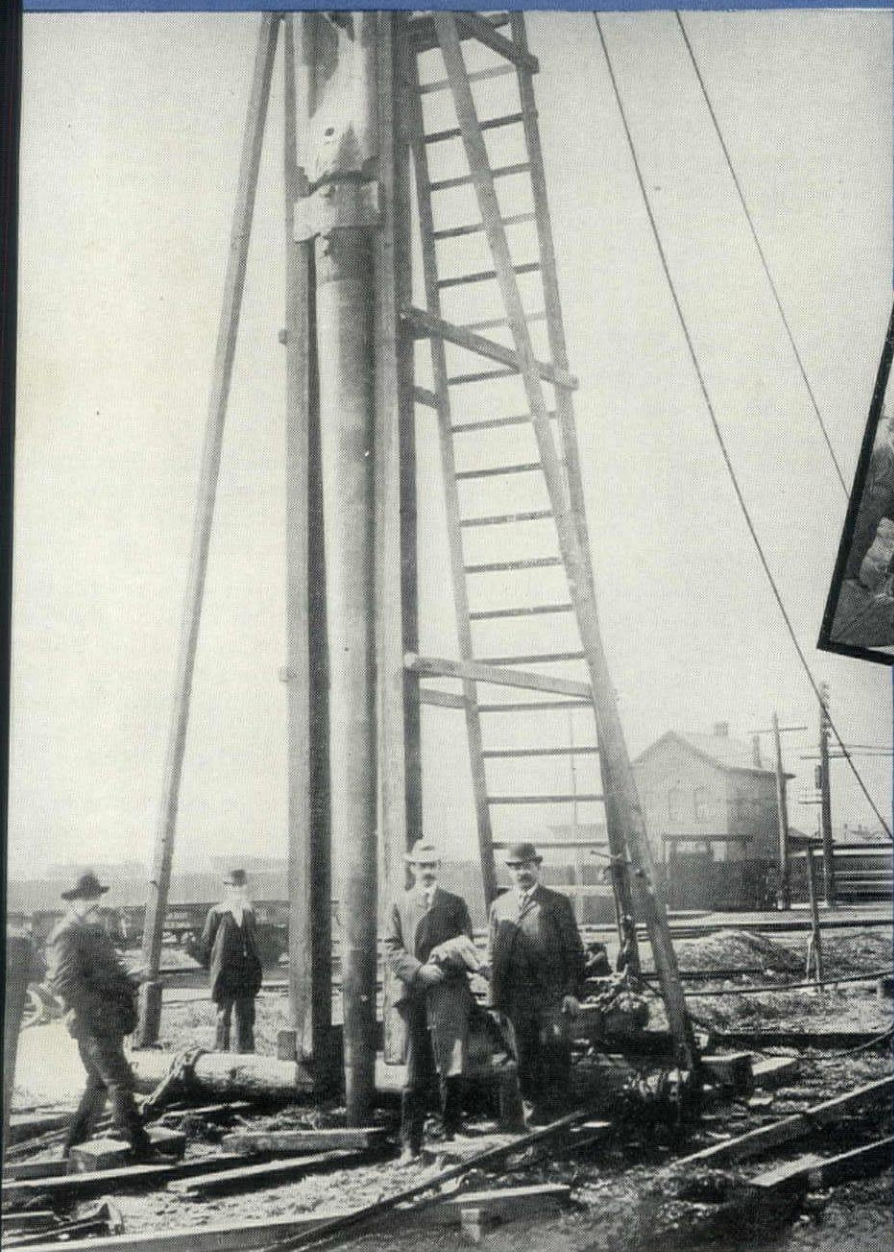
(LEFT)—Mr. A. A. Raymond (wearing derby) supervising the driving of the first Raymond Concrete Pile.
