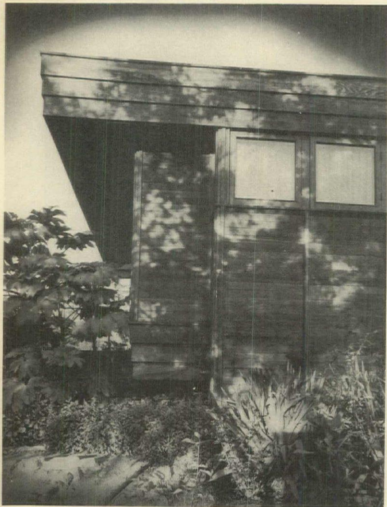
WHERE EAVE IS REQUIRED, HORIZONTAL BAND IS PROJECTED ABOVE WINDOWS
