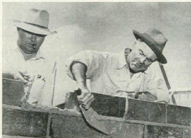
Ricement blocks being laid, builder-manufacturer Hollis with cigar (l), inventor Chappell shows how blocks can be sawed.
