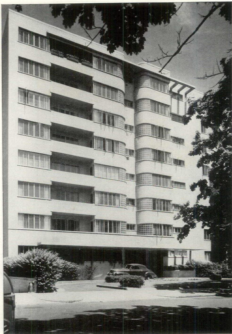
Curved panels of Insulux Glass Block bring daylight with privacy to tenants of eight-story apartment building. Architect: Berla & Abel, Washington, D. C.
