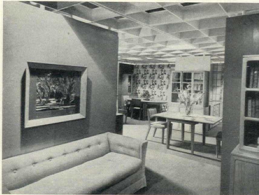
MODULAR CEILING GRID permits great flexibility in placement of partitions.
