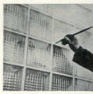
freezes and causes the block to crack. By forming a film over the joint which expands and contracts with the mortar as well as the glass the new material waterproofs the joints. Klee Sealant is of plastic-like consistency, can be applied with a caulking gun or thinned down with solvents to brushing con-(Continued on page 168) sistency. It remains rubbery
