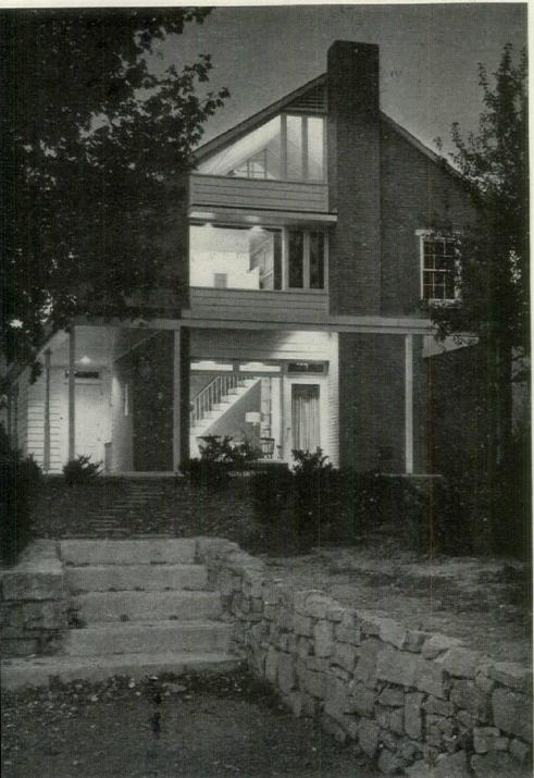
NON-STRUCTURAL BRICK WALL FACING SOUTH WAS REPLACED WITH GLASS
