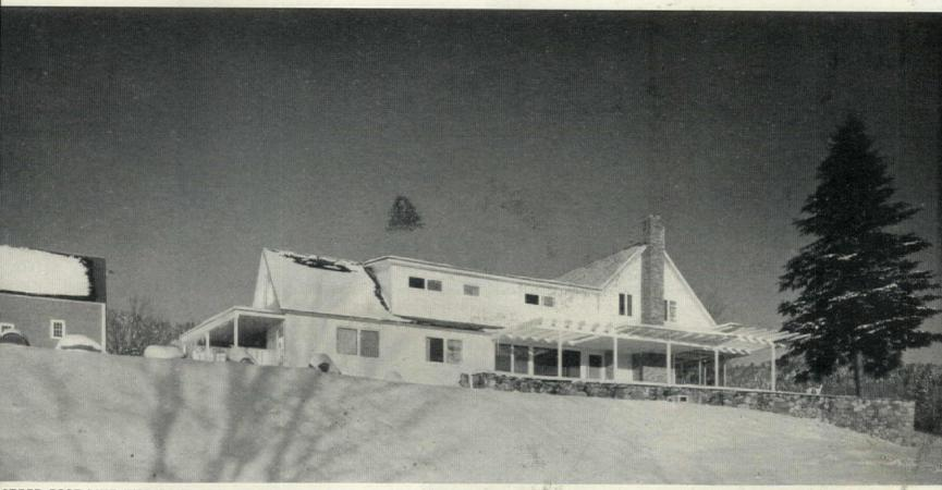
STEEP ROOF LINE WAS BENT AND EXTENDED OVER NEWLY GLASSED FIRST FLOOR WALLS FOR PROTECTION AND SUMMER SUN SHIELD
