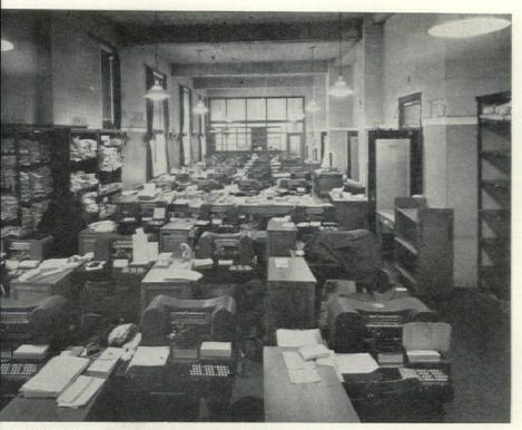
**SAME ROOM**, in the photograph below, is estimated to be 25 per cent more efficient for work-production than in the photograph above, taken before the three stages of illumination redesign, painting, and refinishing were begun.
