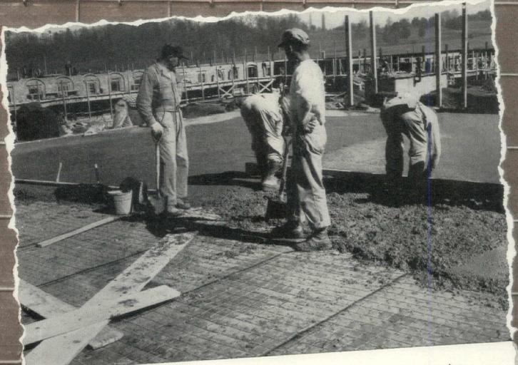
Floors are placed faster with Pittsburgh Steeltex Floor Lath. Additional reinforcement is not required because Steeltex Floor Lath is a combination of form and reinforcement for both concrete and gypsum floors and roofs.
