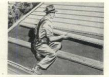
Roofing has all the features of the siding and can be applied at lower cost than shingles.
