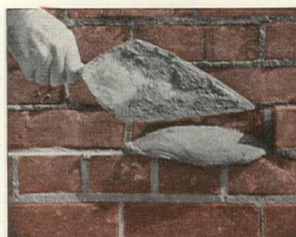
Method 3. A full trowel of mortar should be thrown on the wall.
