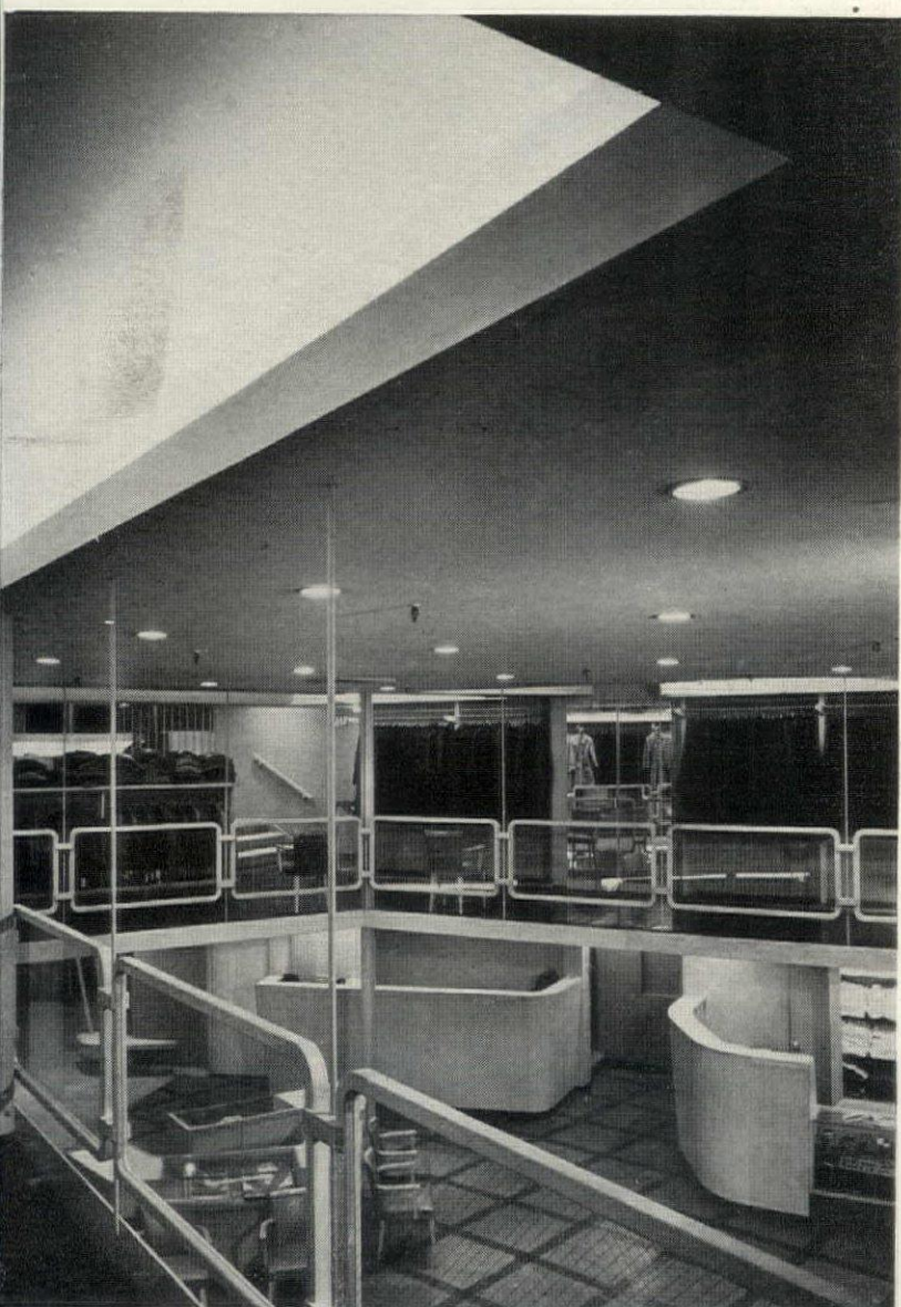
FRAMED PANELS OF WIRED GLASS MAKE UP RAIL OF MEZZANINE
