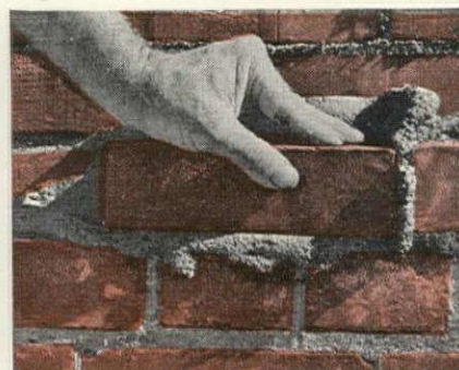
Then the brick should be shoved into this deep bed of mortar.
