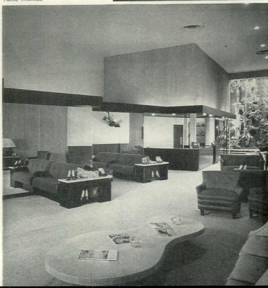
ZIG-ZAG MIRRORED SCREENS CONCEAL STOCKROOM, CARRY LIGHT COVES
