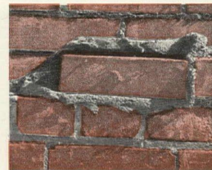
So that the mortar oozes out at the top of the joint.
