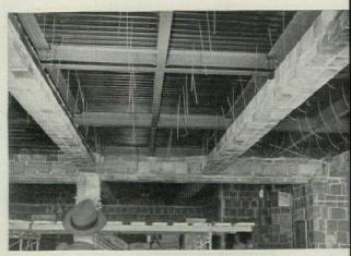
STEEL BEAMS were fireproofed with clay tile before corrugate steel floor deck was sprayed with Limpet asbestos plaster
