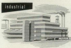
When this new plant for producing "juke boxes" was built, large glass areas were installed to provide plenty of light. The huge windows and the skylighted saw-tooth roof presented a heating problem, but a Trane system cut drafts, reduced wasted heat, and gave workers comfort.
