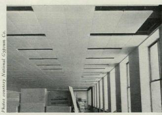
PERFORATED METAL CEILING needs no absorbing pads Sprayed Limpet acts as sound absorbent as well as fireproofing
