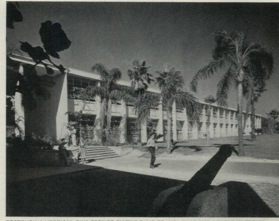
PROTRUDING VERTICAL FINS FORMED BY THE RIGID FRAMES TRAP THE BREEZE IN EDDIES
