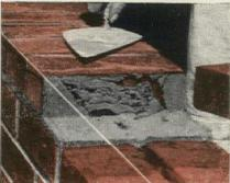
Slushing will not fill the voids.
