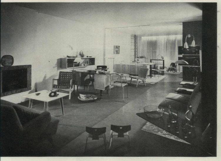
Aside from removing a lot of antiquated plumbing and all non-load-bearing partitions, the transformation of the old kitchen floor was largely a matter of new surfaces. The floors are a reddish-brown oak chip and plastic cement compound, laid on metal lath over the old wood flooring. The walls are of whitewashed brick, white and light gray plaster, walnut plywood and a South Seas grass cloth. Street windows are curtained in sheer white, those of the bay at the rear in chartreuse.
