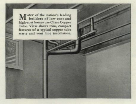
Past... economical installation has made Chase Copper Tube for soil, waste and vent lines a favorite with builders coast-to-coast! Here's why: You reduce many connections because Chase tube is available in 20 foot lengths. Its light weight makes pre-cutting and pre-assembly possible... makes maneuvering and handling quicker!
