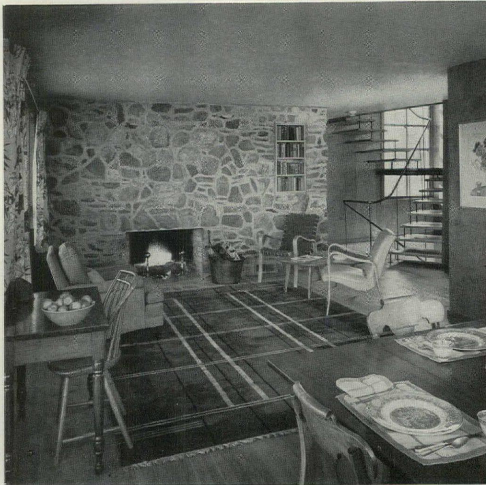
MASSIVE MASONRY CORE EXTENDS UPWARD THROUGH HOUSE, FOR FURNACE FLUE AND FIREPLACES IN STUDY, LIVING ROOM AND PLAYROOM
