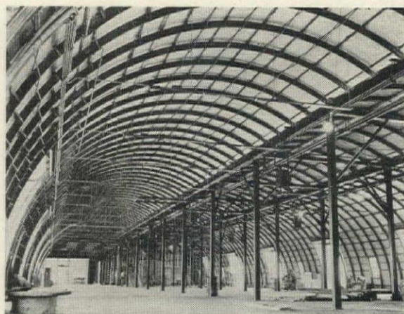
Outbound cargo building interior shows Spraykote insulation applied to steel-ribbed walls.
