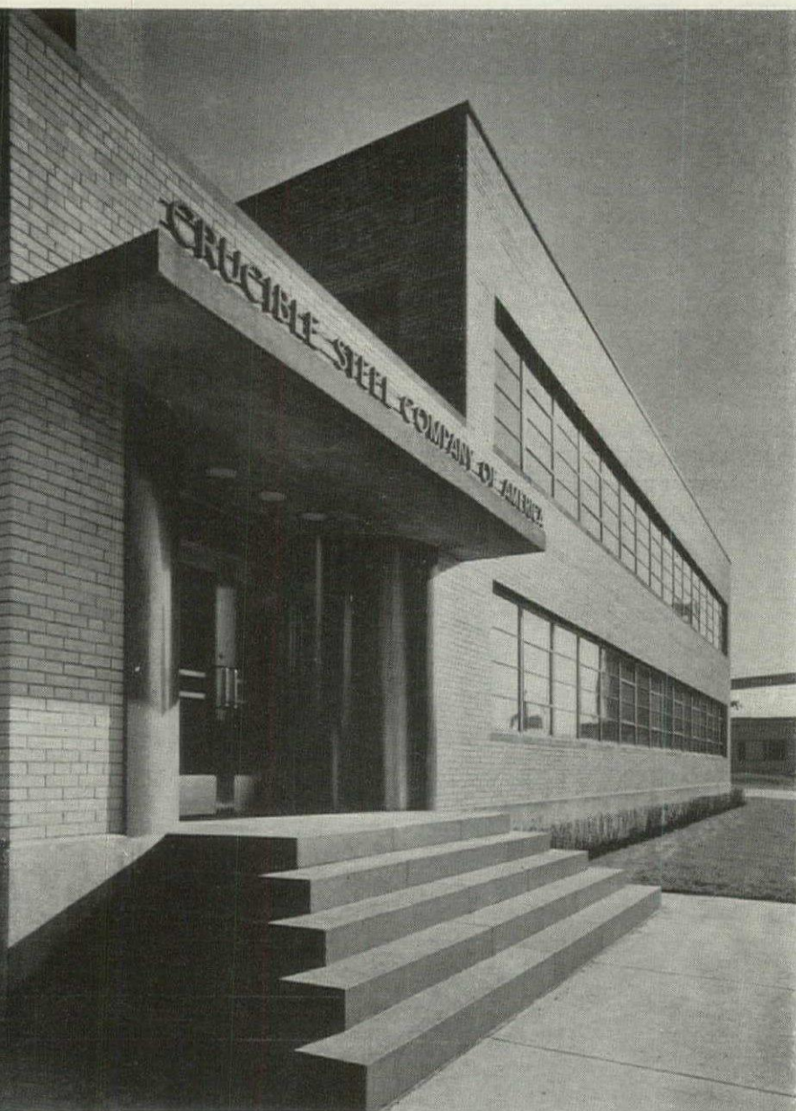
MAIN ENTRANCE; THE STRUCTURE IS STEEL, BRICK ENCLOSED
