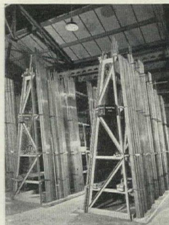
VERTICAL STACKING of steel is innovation, simplifying handling by crane from above. Warehouse floor is concrete, with heavy reinforcing and special hardening agent.
