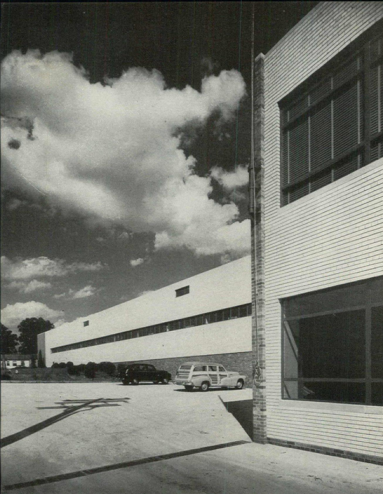
WEATHERED HORIZONTAL MASONRY JOINTS GIVE STRONG TEXTURE TO BUFF BRICK WORK
