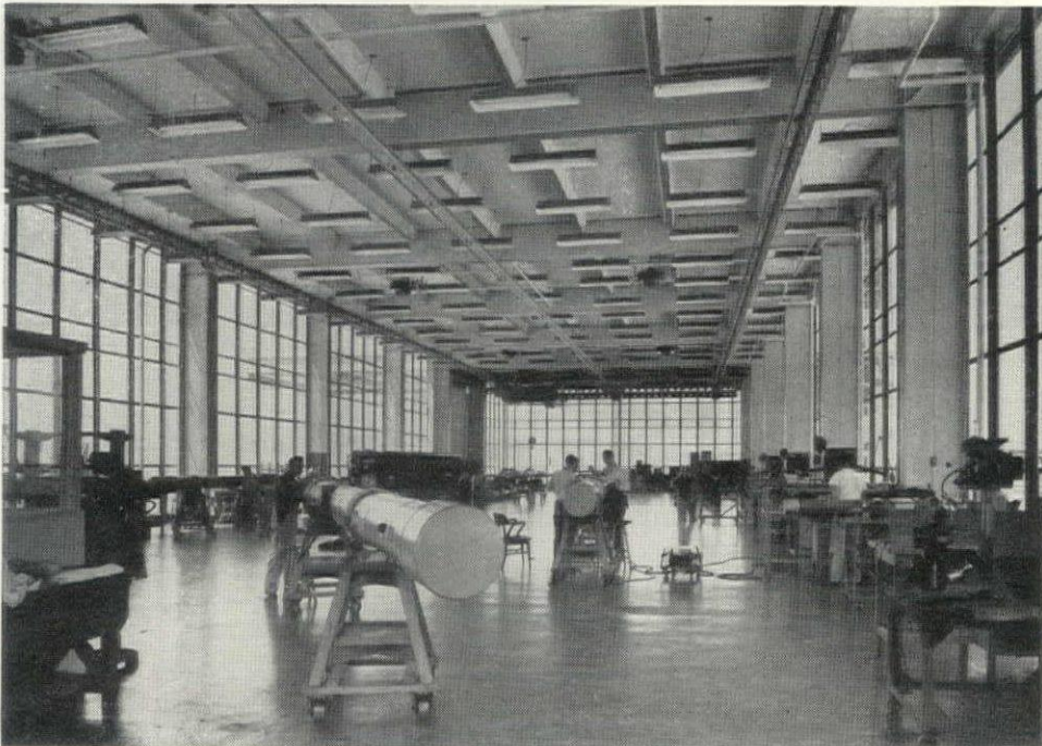
PERISCOPES AND RANGE FINDERS ARE CALIBRATED, REPAIRED IN OPTICAL SHOP
