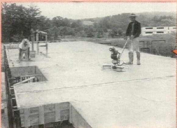
Two-inch concrete floor has been poured and finishing operations are under way.
