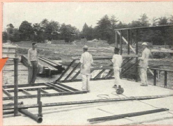
Raising a precision Stran-Steel wall panel into position.
