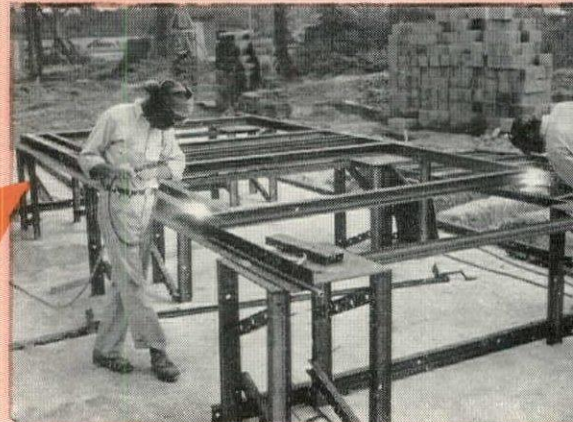
Accurately-sized Stran-Steel studs are now assembled into wall sections.
