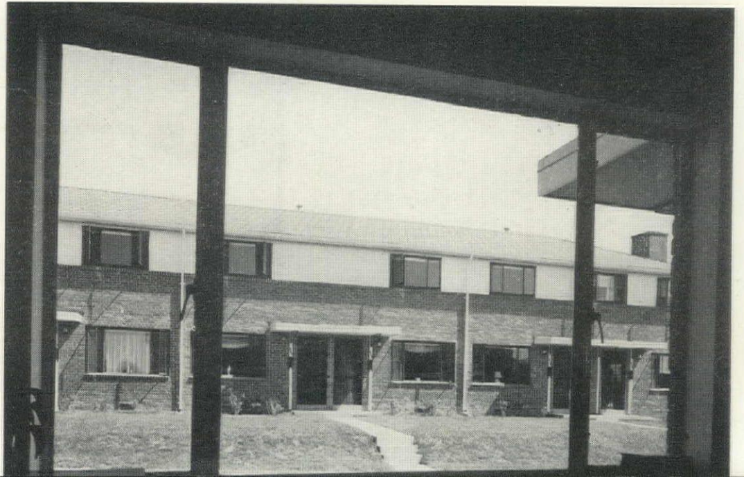
BRICK-VENEER CONSTRUCTION STANDARD IN AREA IS ENLIVENED BY ASBESTOS SIDING
