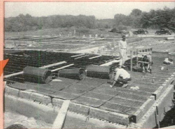
Fibre-backed steel mesh is nailed directly to Stran-Steel joists.
