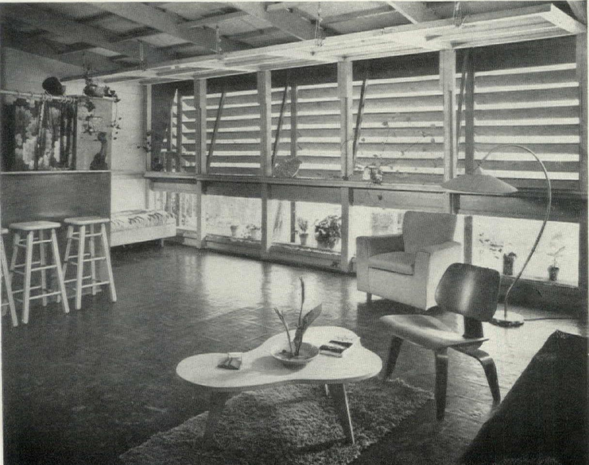
LIKE THE EXTERIOR, THE INTERIOR LEAVES STRUCTURE EXPOSED. NOTE PULLEY-OPERATED WINDOW
