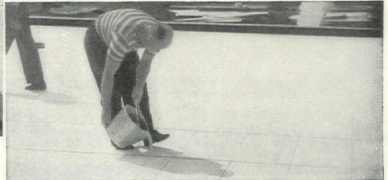
WHEN American Structural sub-purlins are used, insulating grout, shown above, provides necessary anchorage by gripping the stem of the sub-purlin. Through the use of bent studs, Kaylo Roof Tile can be applied directly to trussed purlins or standard shapes without the use of sub-purlins, as shown in the drawing below.
