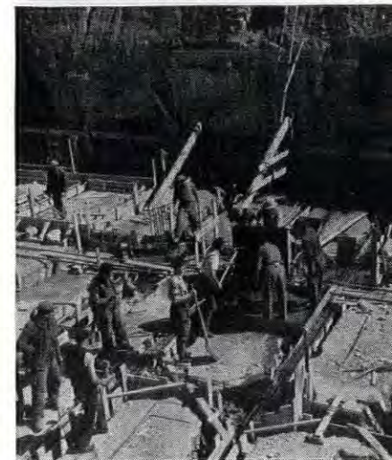
REINFORCED CONCRETE replaces old type masonry in French reconstruction. Scarcity and high cost of materials has slowed many projects. In spite of this, France has plans for 1,615 of its 1,900 damaged cities.
